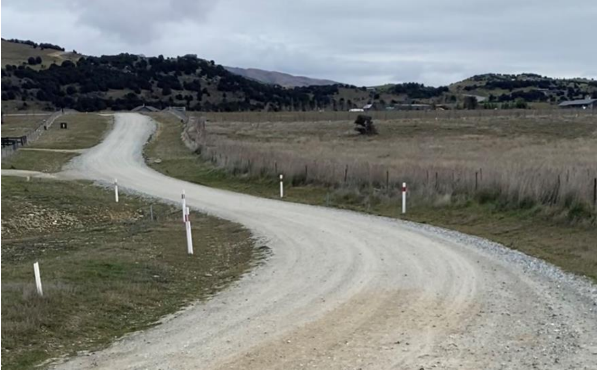
Figure 1.6 Culvert with reflector edge markers.
