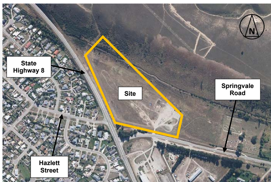
Figure 2: Aerial Photograph of Site and Environs
