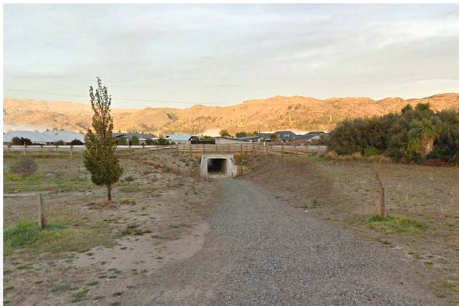
Photograph 7: Underpass below State Highway 8
