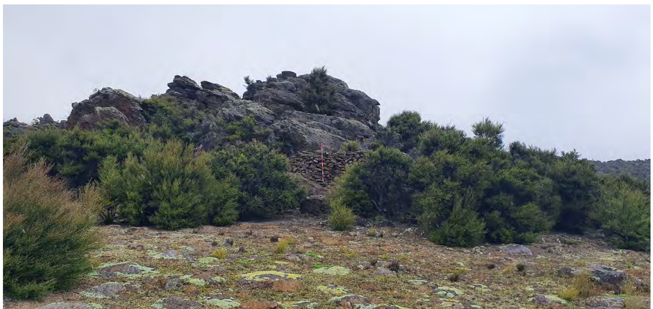
Figure 2. Photograph of G41/772 retaining wall from NZTM E1308011 N5017234, facing south.
