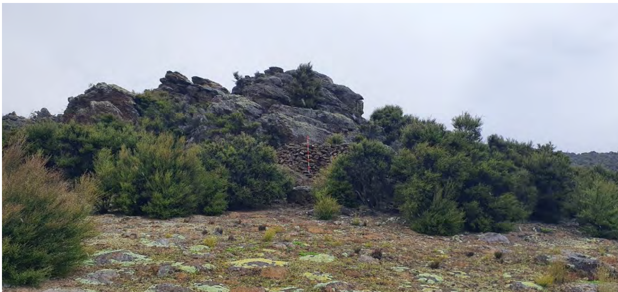
Figure 13. Photograph of G41/772 retaining wall from NZTM E1308011 N5017234, facing south.
