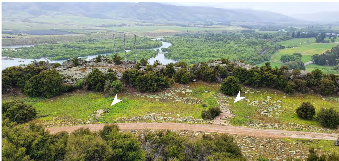
Figure 2. Site 4 from NZTM E1308223 N5017420, facing north. Arrows show banks and point to locations where revetting is present.
