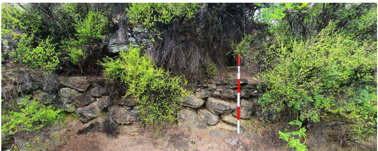
Figure 16. Lower section of wall at southern end.
