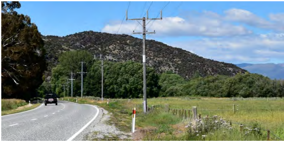
View Looking South the 'Elevated Rock Knoll' from SH8
