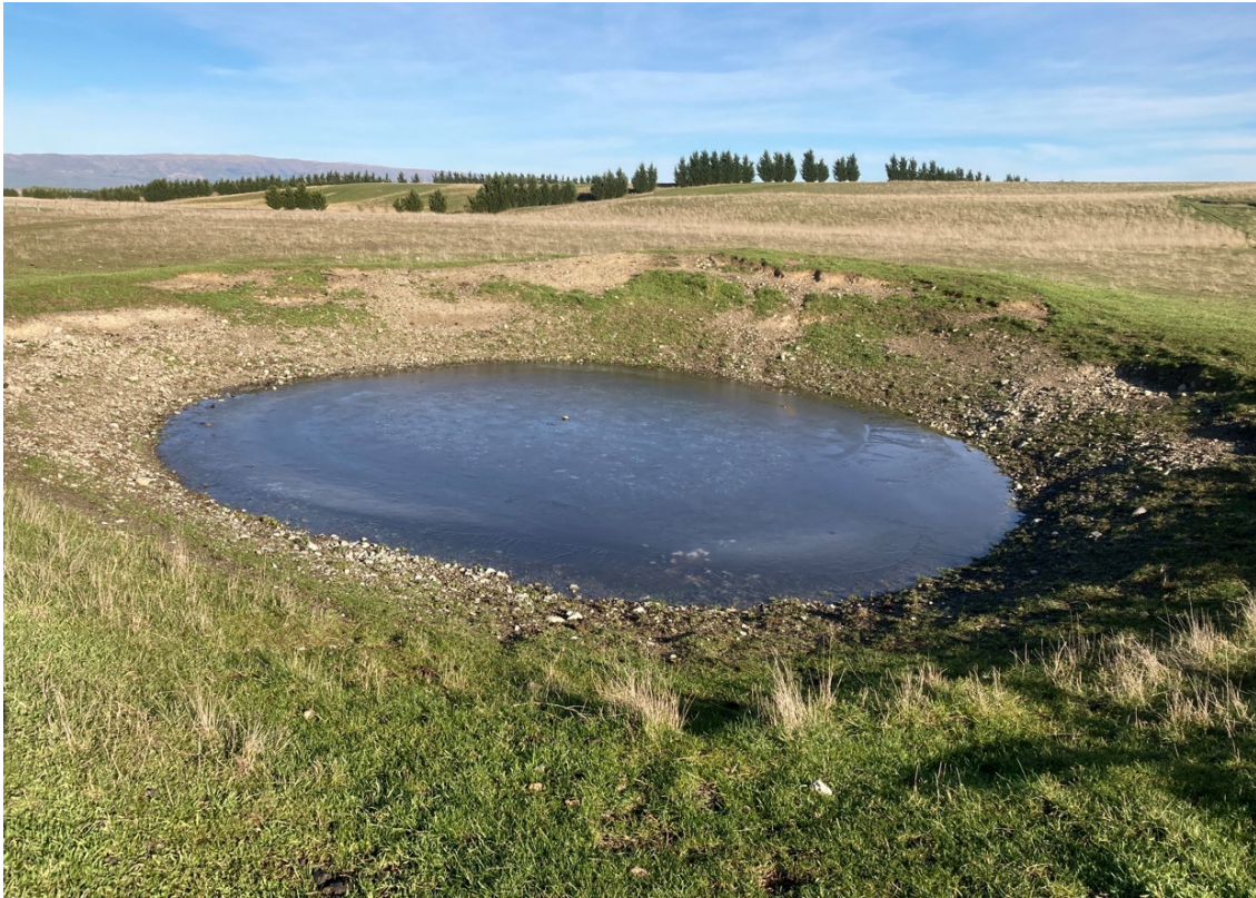
Figure 12. Constructed pond, showing evidence of excavation and bunding from historic earthworks.
