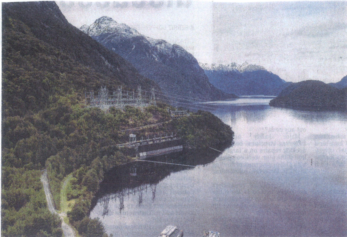
Filling up . . . Meridian Energy's Manapōuri power station.
