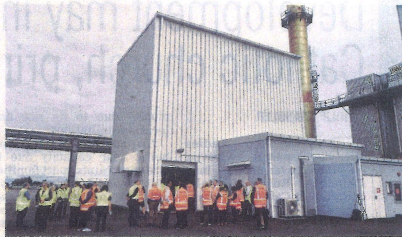
Unveiling ... The new electric boiler plant at Fonterra Edendale.
