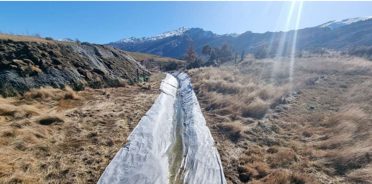
The standard GD05 design with a trapezoidal shape with a 100mm base width and a height of 550mm (250mm + 300mm freeboard) with 2:1 side slope.
