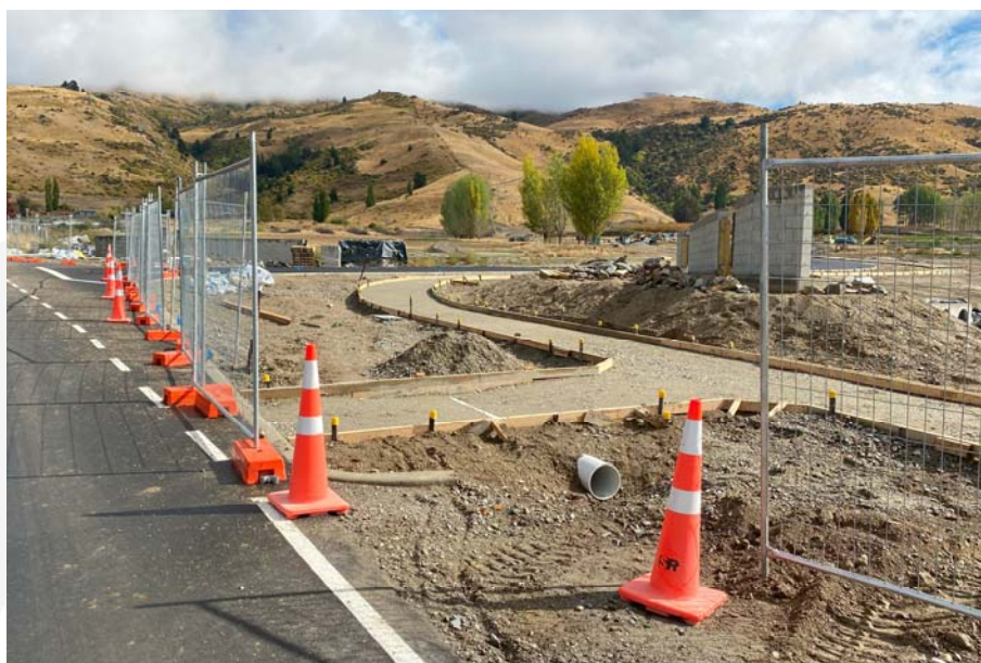
Photograph 6: Shared Walking and Cycling Route Alongside Ripponvale Road
