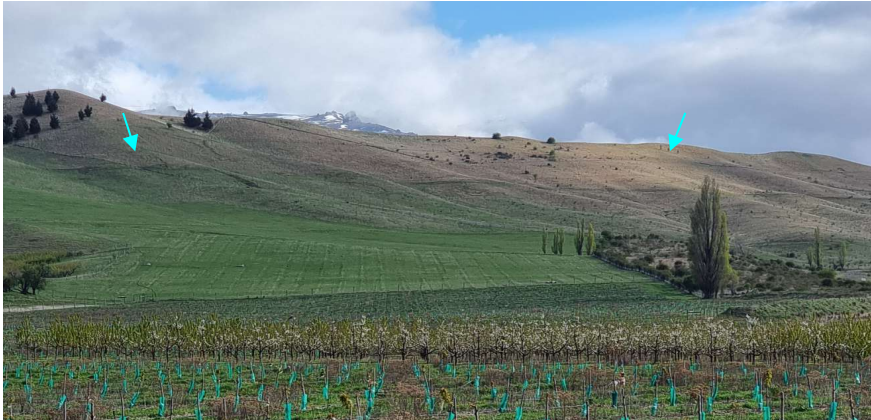
Example of stabilised existing water races on site. These will be utilised to capture upslope overland flows and divert around works areas. Where it's not possible to utilise the existing water races, GD05 design clean water diversions should be installed.
