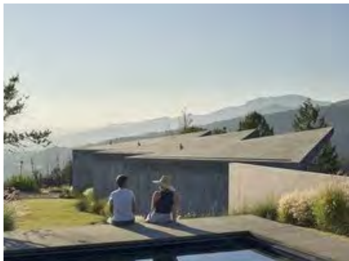
Figure 5. Mono-pitch roof addresses hill slope
