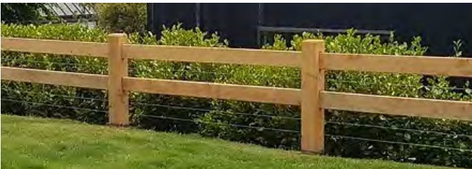
Figure 11. Post and rail fence
