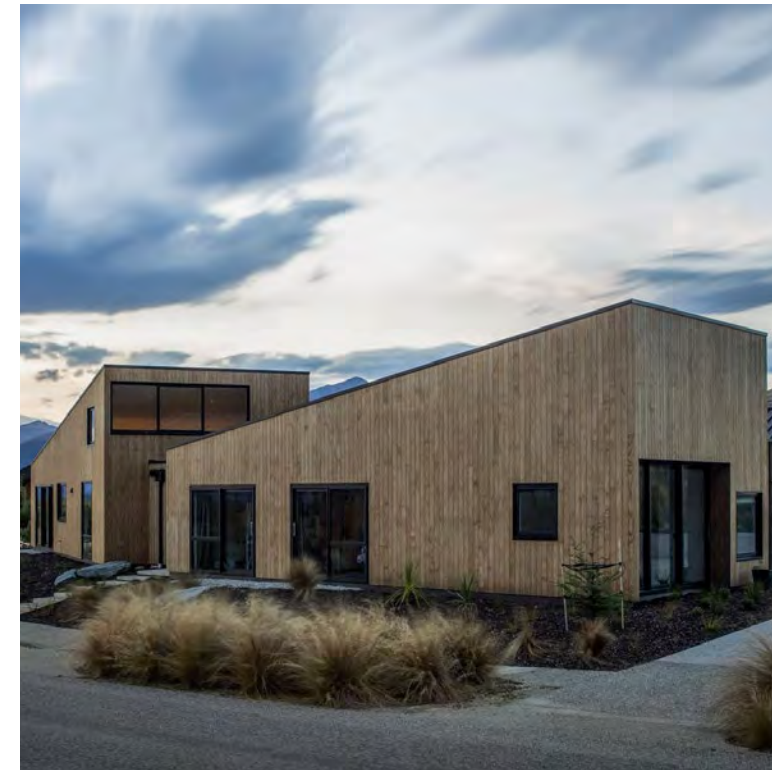
Figure 8. Jacks Point home by Ben Hudson Architects
