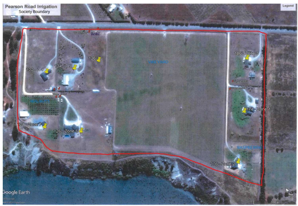
Figure 9: Properties serviced by the PRIS (Image Source: PRIS Water Safety Plan).
