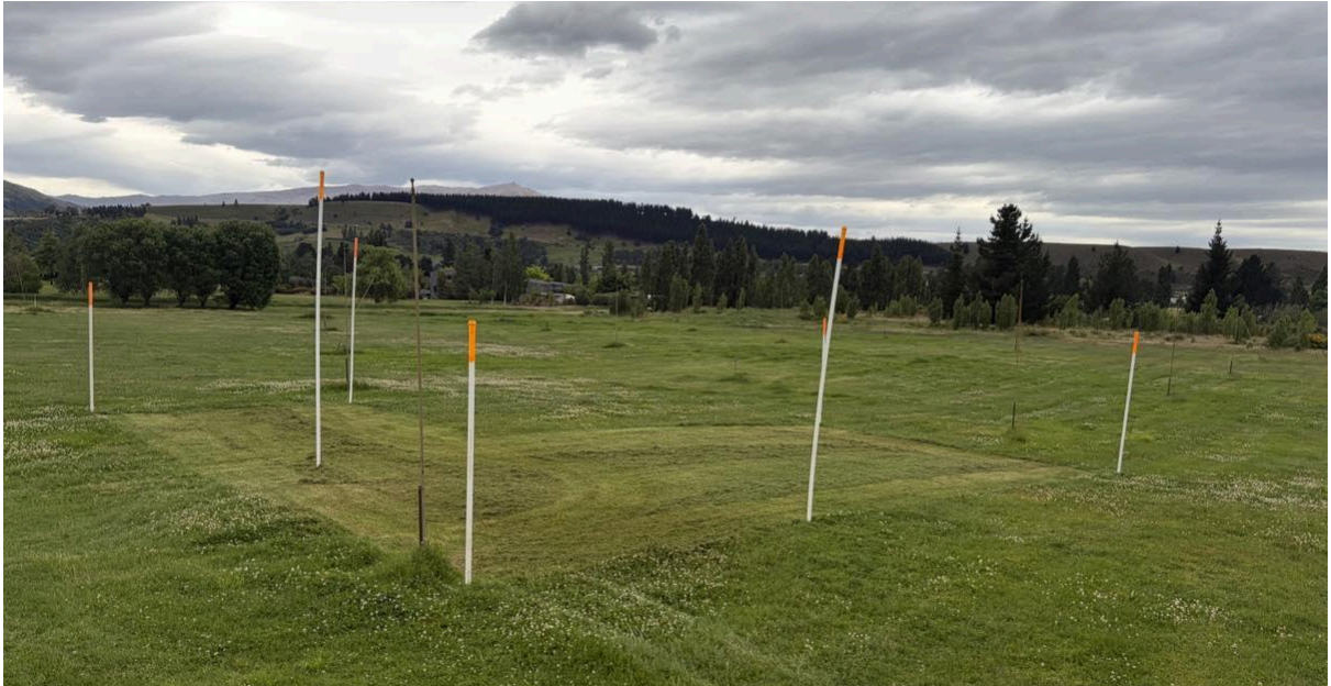
Figure 2 - Profile poles on site (refer plans for reference)
