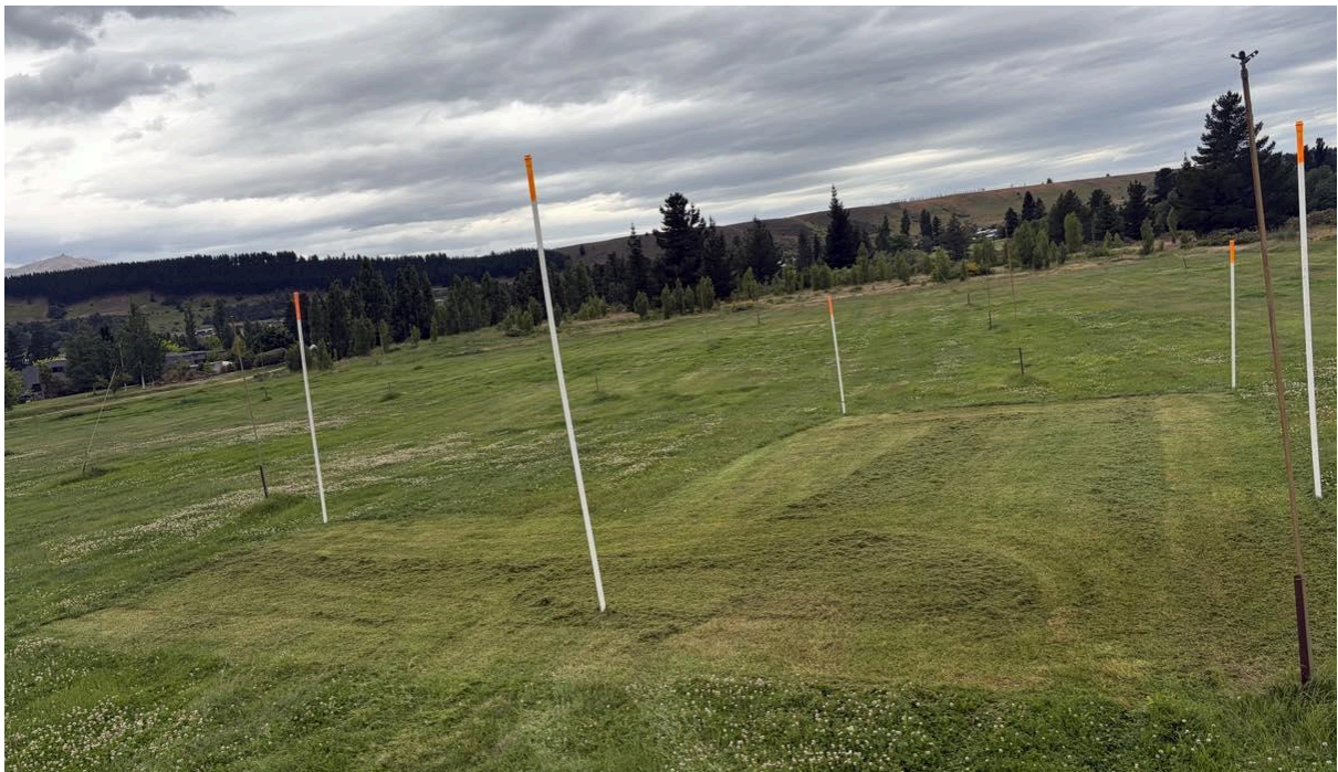
Figure 1 - Profile poles on site (refer plans for reference)
