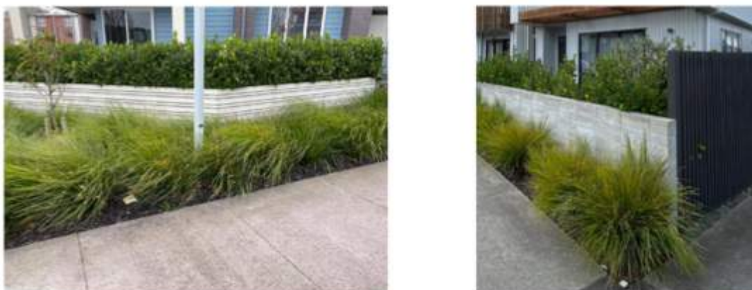
Figure 2: Imagery – Streetfront Wall & Planting
