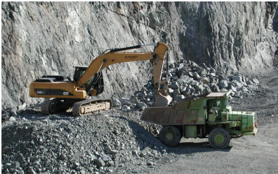
Figure 2. Cat 330D Excavator
