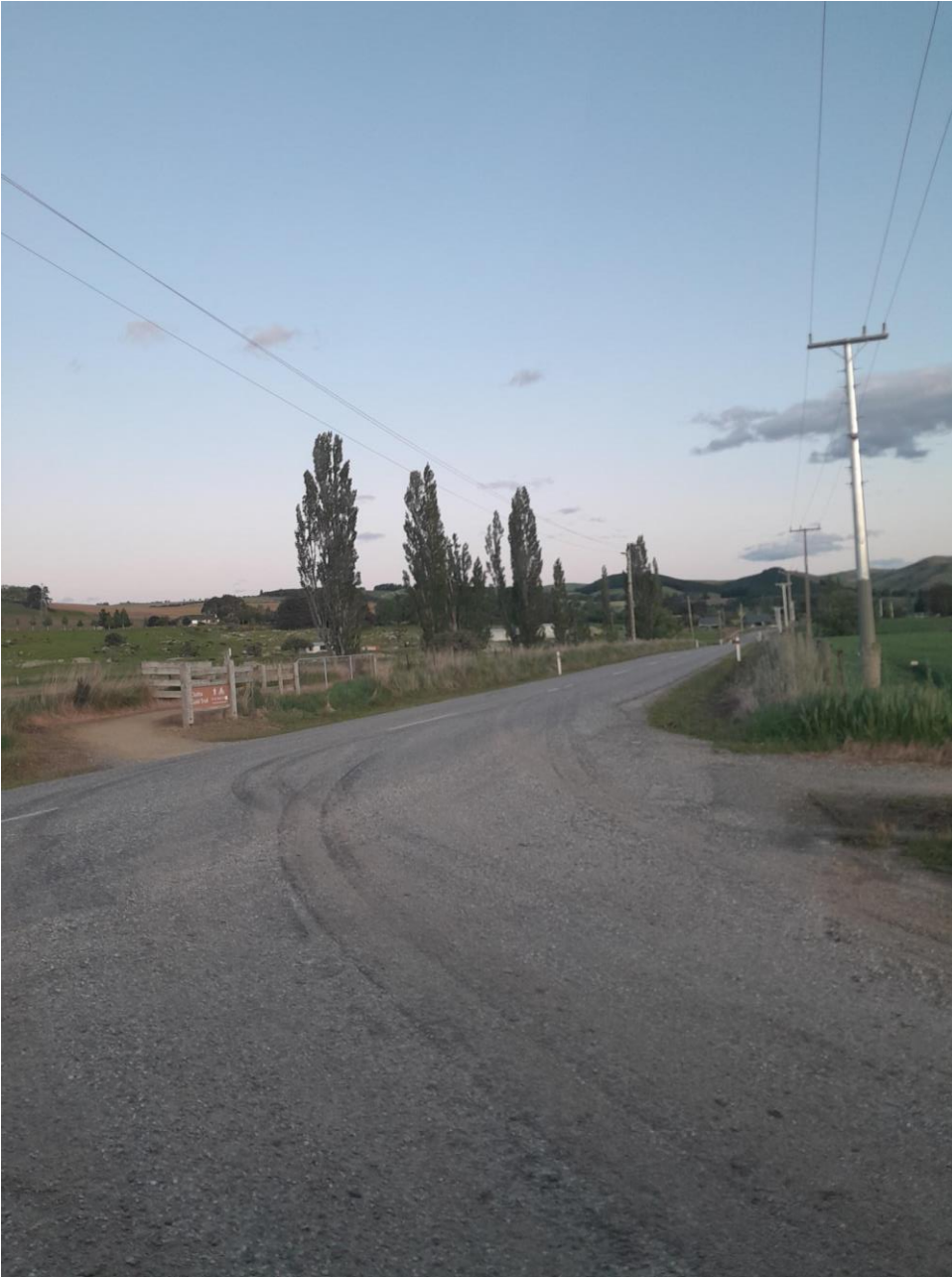
Figure 4.2 Looking south-east from southern access
