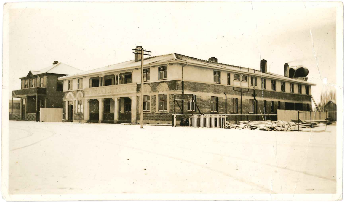
Ranfurly Hotel. Geoffrey helped wire the new annex at right. The building replaces the one burnt down. He points out that the foreground is snow not sand.
