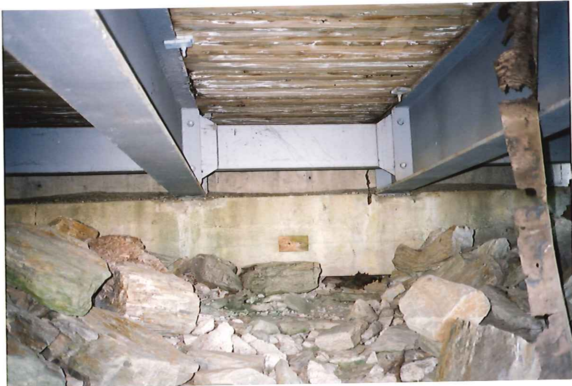
Description: View under at TL abutment
