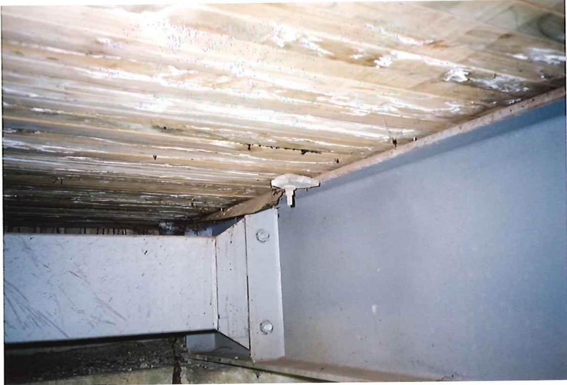
Description: Typical decking fixing
