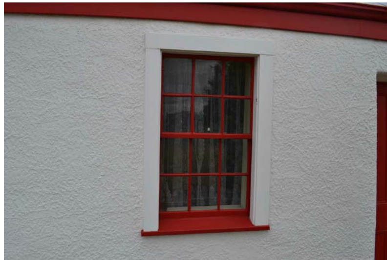
5. Window W1 (left of the front door) - 6 over 6 sliding sash
