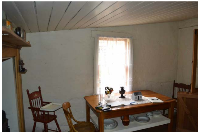
4. Room 4 showing the paint finished plastered mudbrick walls and window on the east wall.
