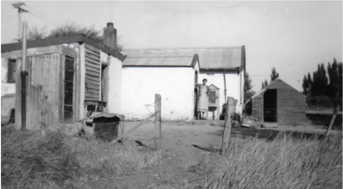
Figure 25 The rear of the cottage with the timber sleep-out (right) and wash house and corrugate clad WC (left). Photograph: Courtesy of the Vallance Family Records
