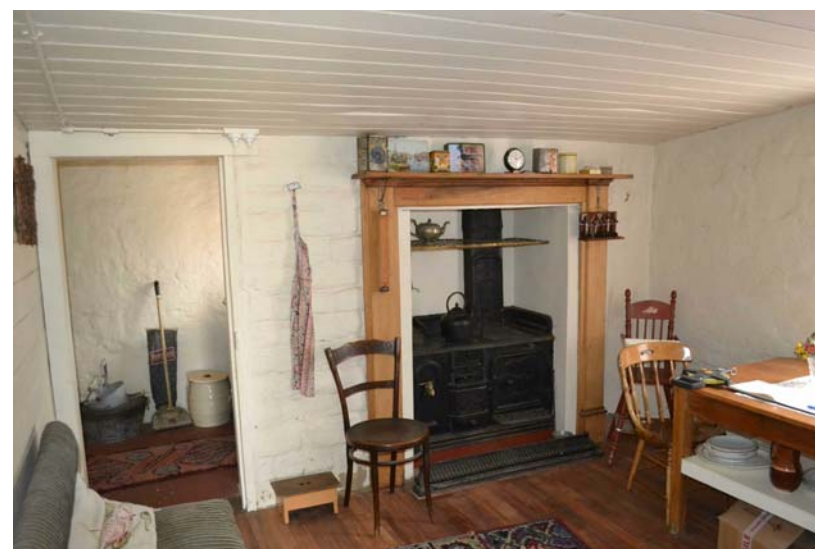
5. Room 4 showing the mono-pitch t&G ceiling and shacklock range with timber mantel. Note the different wall types on either side of the range. Unplastered painted mudbrick to the left and paint and plastered mudbrick on the right.
