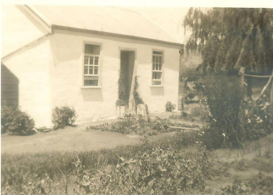
Figure 28 The front of the cottage with grassed garden and flower beds and the timber sleep-out on the left. Photograph: Courtesy of the Vallance Family Records
