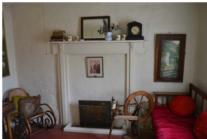
4. Room 2 east wall has a timber mantel and no fireplace.
