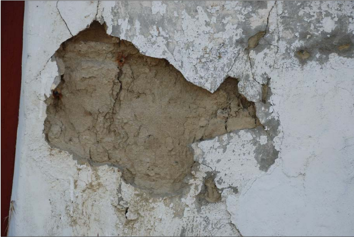
Figure 20: Like Vallance Cottage, the front wall of Peyton's Patch was finished with painted, rough-cast cement render. The side walls however retained their older, smooth render with lime-wash evident beneath the latter paint finish. The photograph shows a section of one side wall where the cracked smooth render had fallen away revealing cob or rammed earth as the principal wall material. Photograph: Origin Consultants
