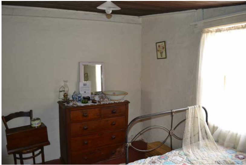
1. Room 3 showing the paint finished plastered mudbrick walls.
