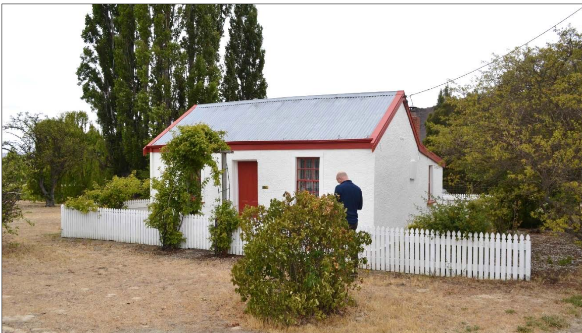
Figure 1: Vallance Cottage in February 2016. Photo: Origin Consultants
