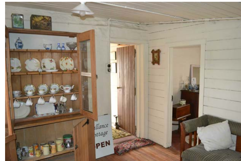
6. Room 4 looking towards the hallway and room 3. Horizontal boarding lines the internal wall adjoining room 3.
