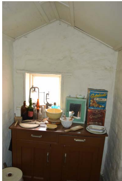
4. Room 6 looking towards the window on the west wall, showing plastered mudbrick wall.
