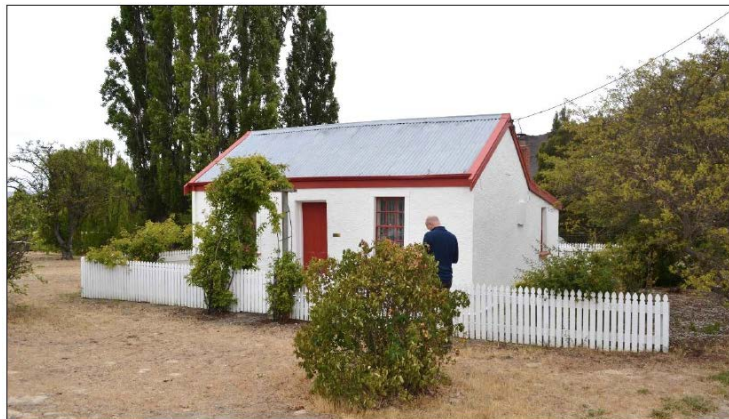
Figure 1: Vallance Cottage in February 2016. Photo: Origin Consultants
