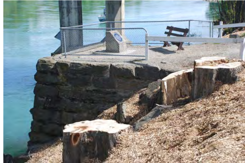
The North Abutment
