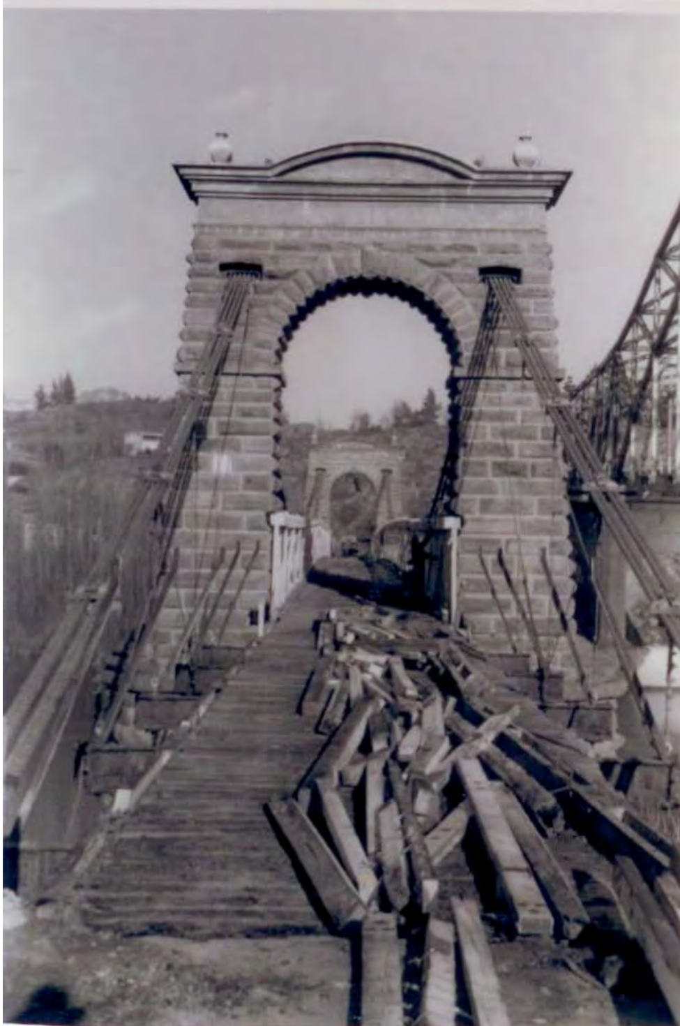
Figure 15 Dismantling the old bridge in 1963 Courtesy of Central Stories Museum
