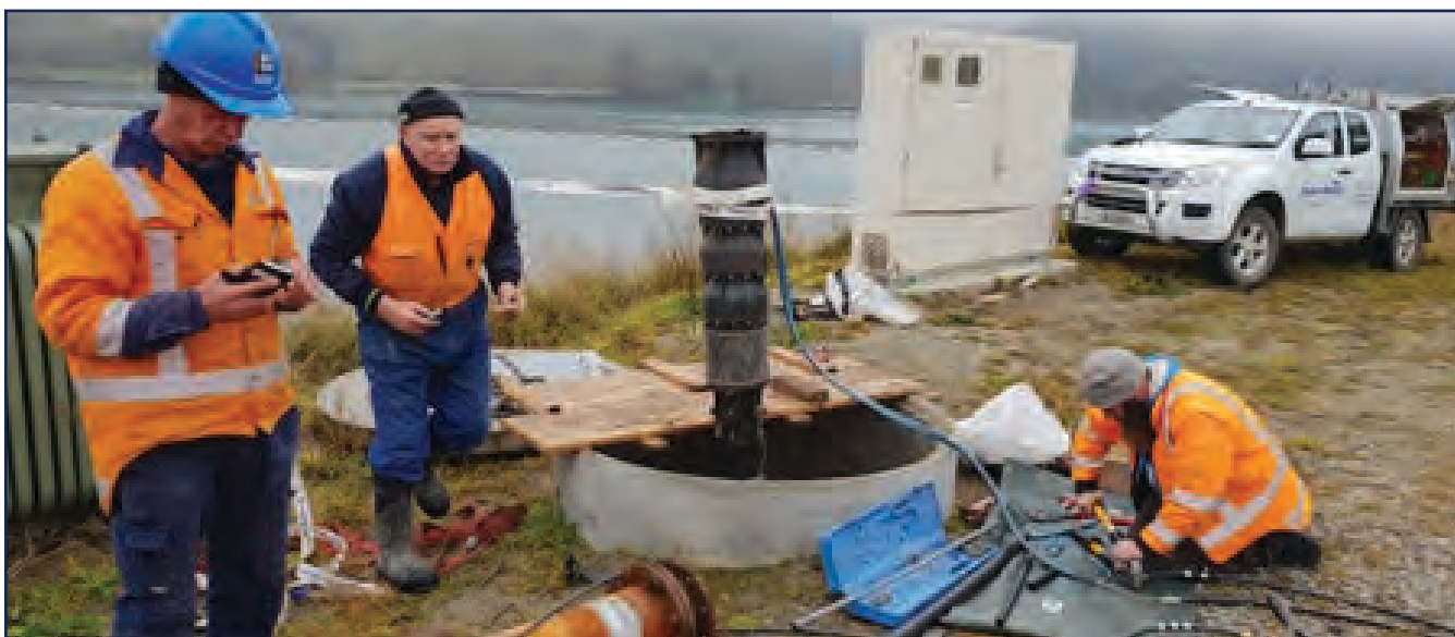
Connecting the spare pump
