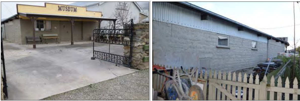
Figure 24: The museum entrance (left) from Fraser Street and the south-west mud brick elevation (right).
