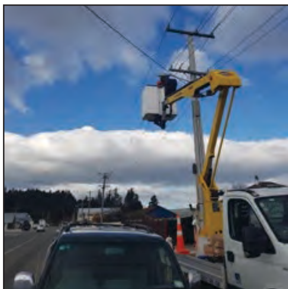
Delta replacing LED light on Station Road, Alexandra – September 2018
