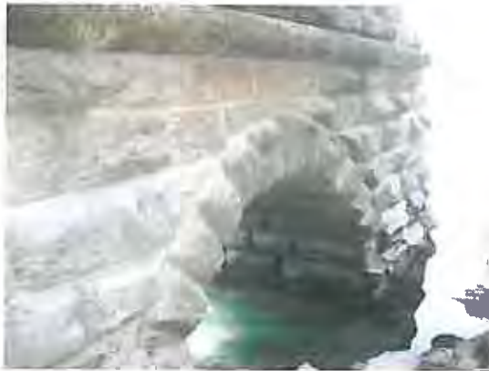
Typical view of masonry in exterior faces of the south pier
