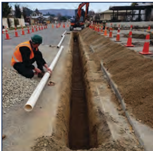
New pipes being prepared for installation on Arnott St
