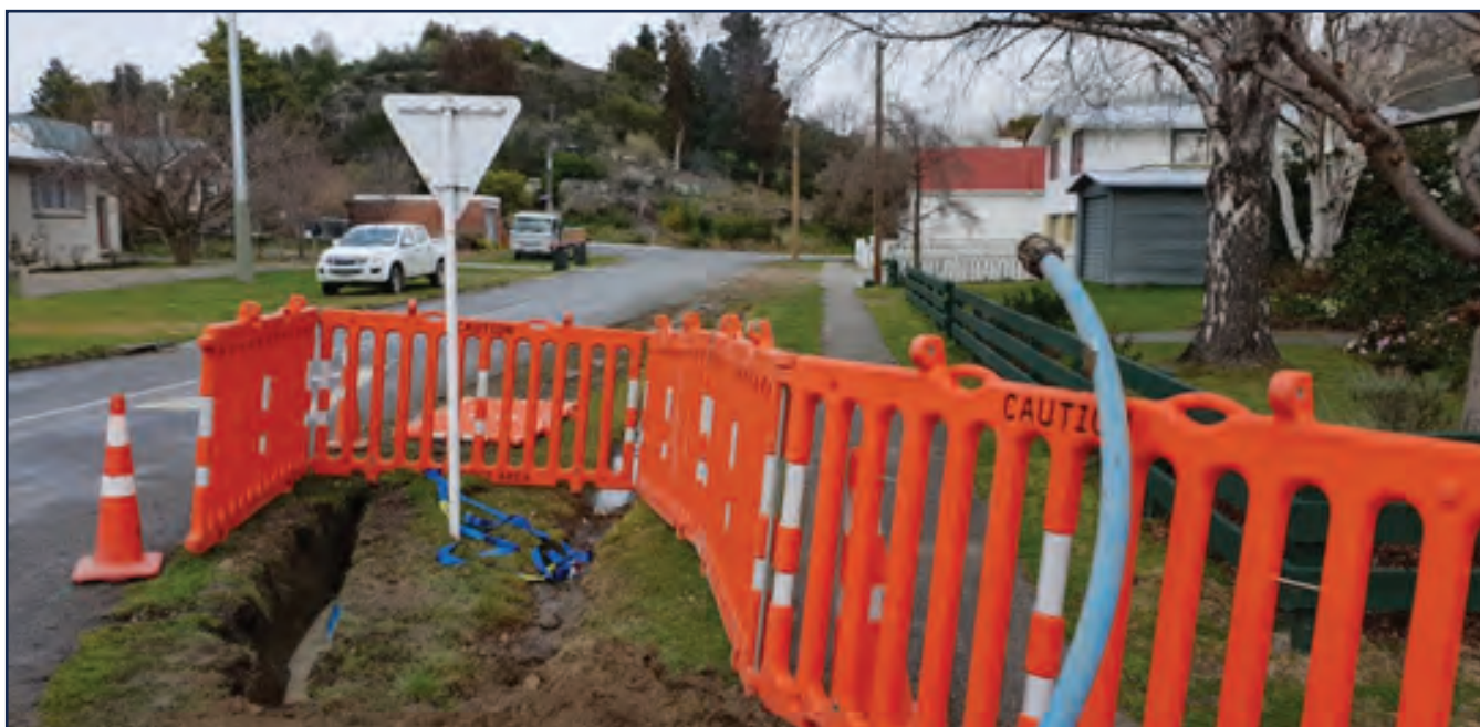
Meter separations being undertaken on Hermitage Street
