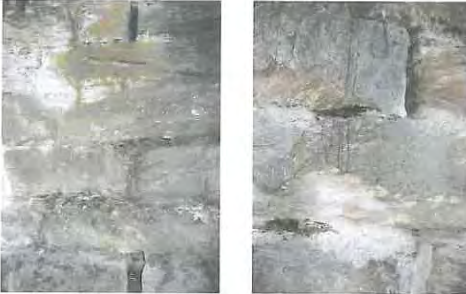
Slots between blocks in front face of Alexandra abutment
