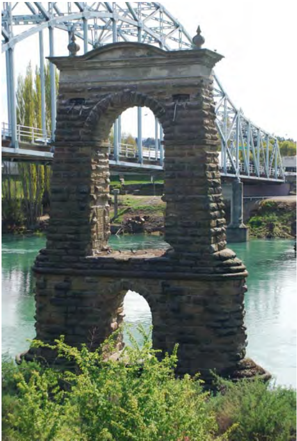
The South Pier and Tower
