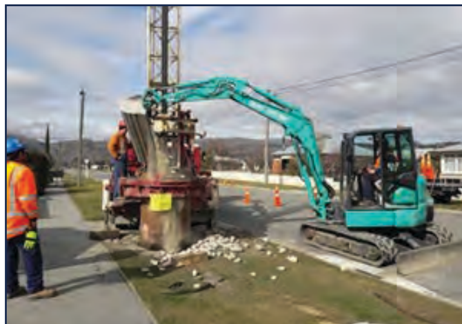
Ventry Street soakpit installation – September 2018
