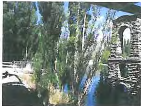
North pier location
