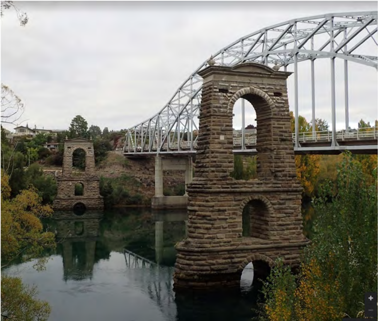
Figure 3. Stone Piers looking South
