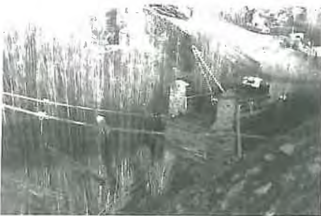
Historical photo of intermediate pier. Note former masonry pillars on each side of pier.
