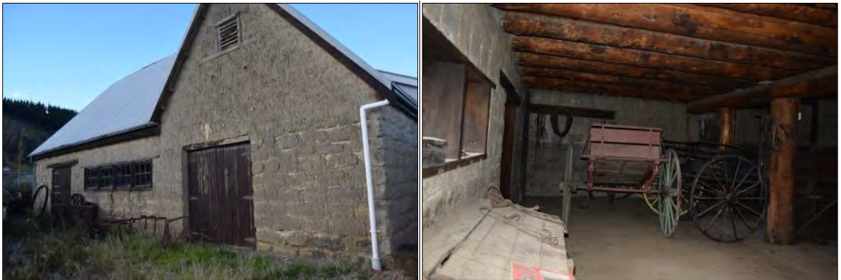
Figure 27: The Stable north-west facing front elevation (left) and interior view of the horse stalls and carriages in store (right).
