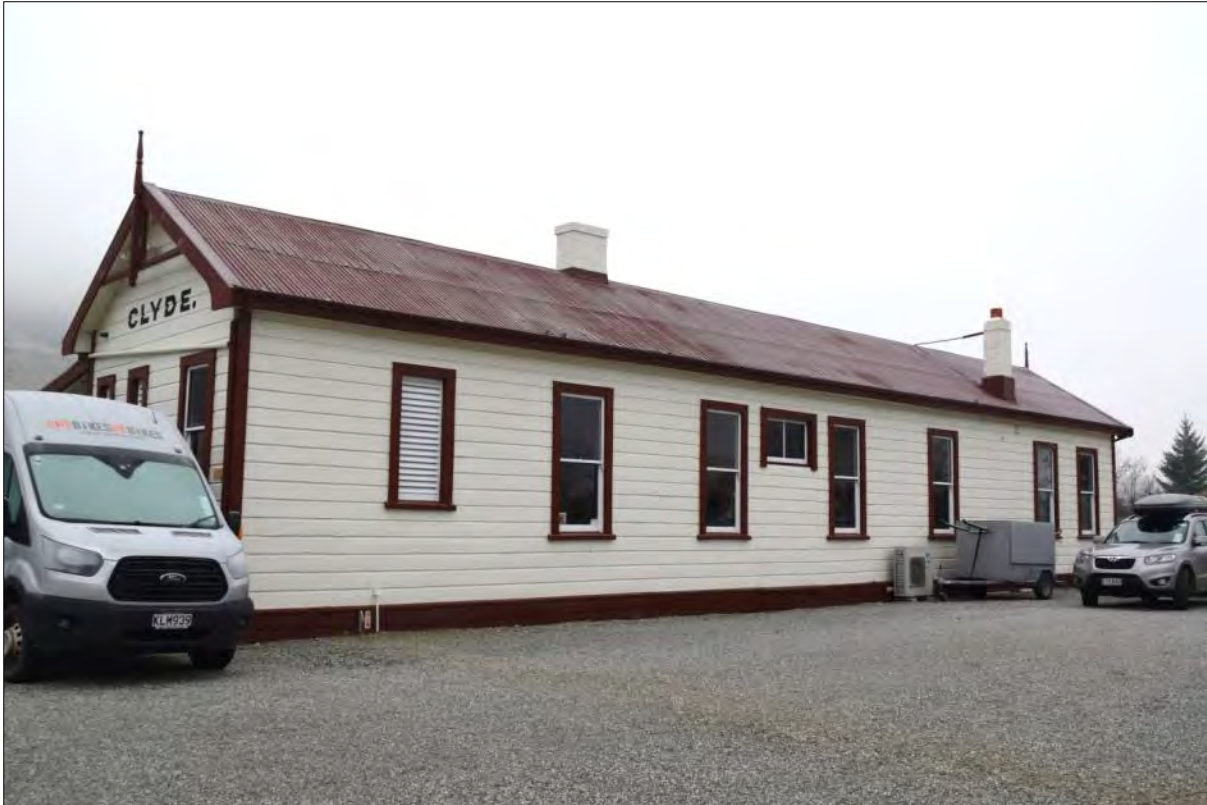
Figure 15: The rear elevation of the station facing onto the car park.
