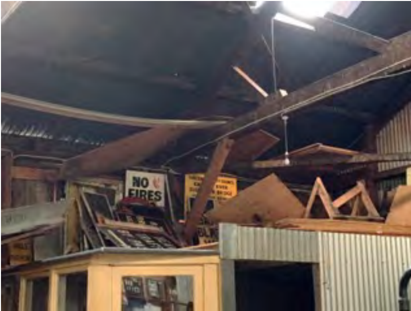
Image: Storage area above the smoko room, as surveyed.
