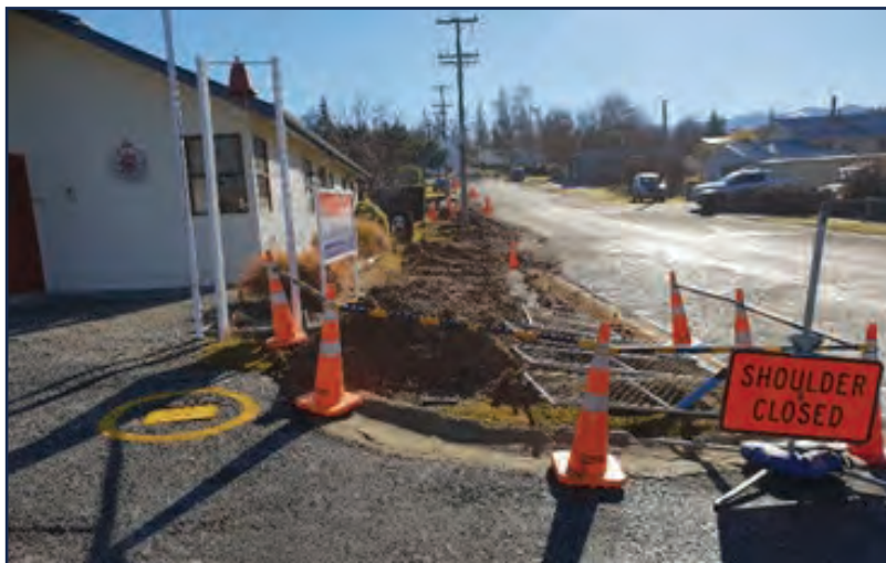
Excavation on Tay St, Naseby
