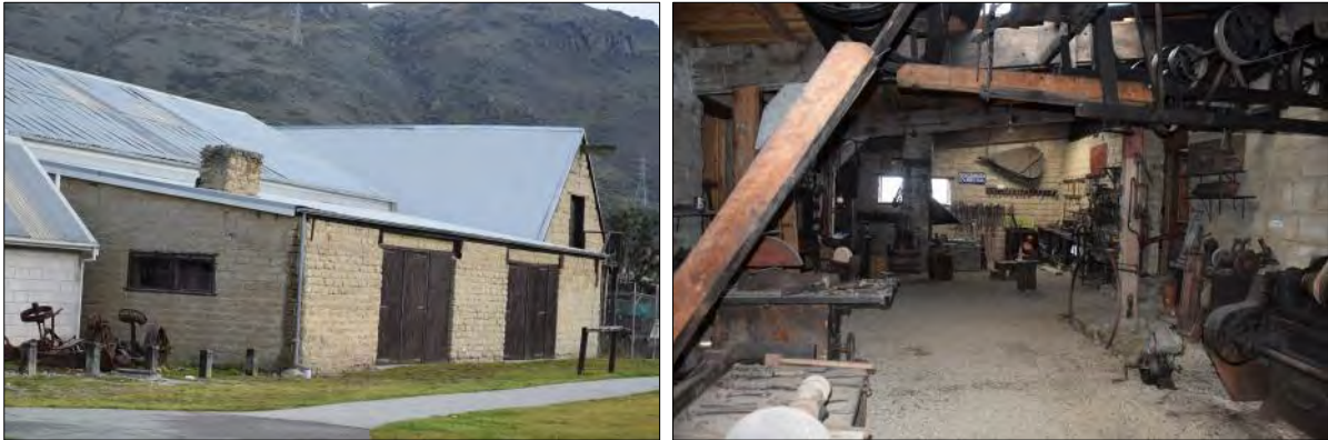
Figure 26: The Blacksmiths building exterior (left) and an interior view looking east (right).
