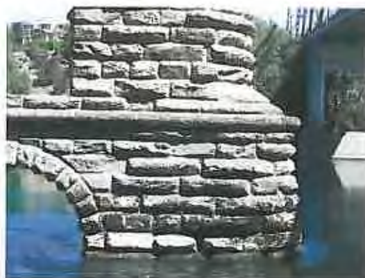
Typical view of masonry in north pier
