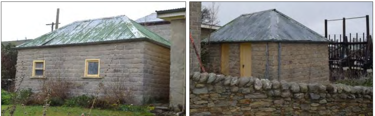
Figure 32: The Dairy building south-west facing exterior (left) and the north-facing exterior (right) with the stamper battery in view in the background.
