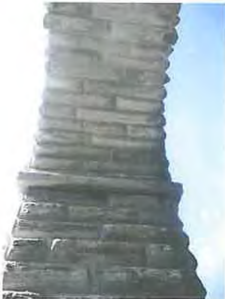
Intrados of upper arch
