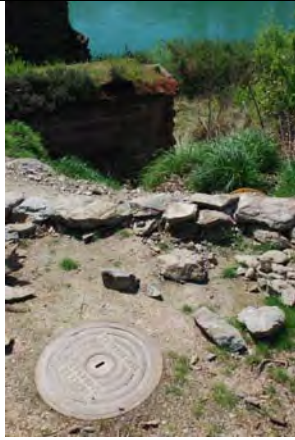
Inspection chamber constructed above the anchorages
