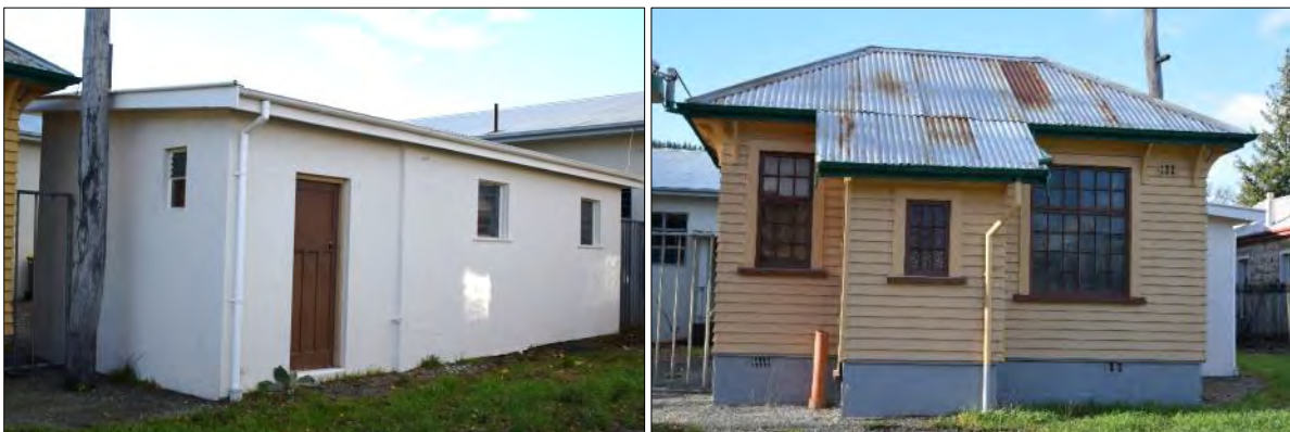
Figure 10: The Ablution Block (left) and Police Lock-up (right) at the rear of the main museum building.
