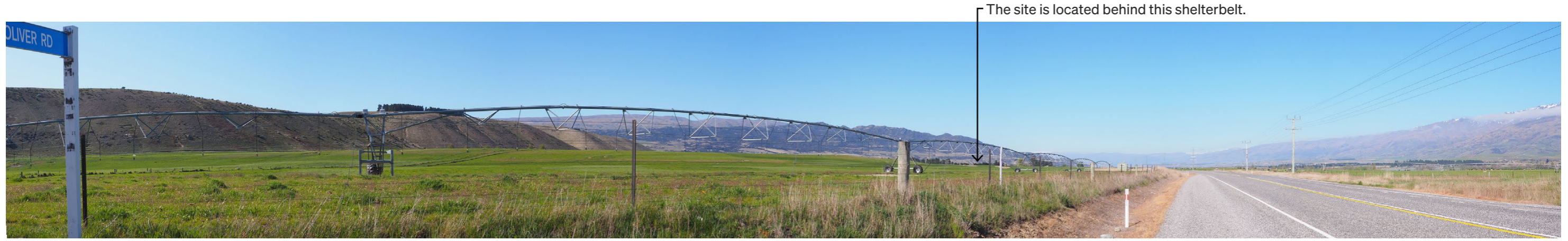
Viewpoint Location Photograph 1: Located at the intersection of SH8 and Oliver Road. The photograph represents the view to the south from this stretch of SH8 and Oliver Road towards the site and its surrounds. Date: 14 October 2022 Time: Between 9:00am and 11:00am.
