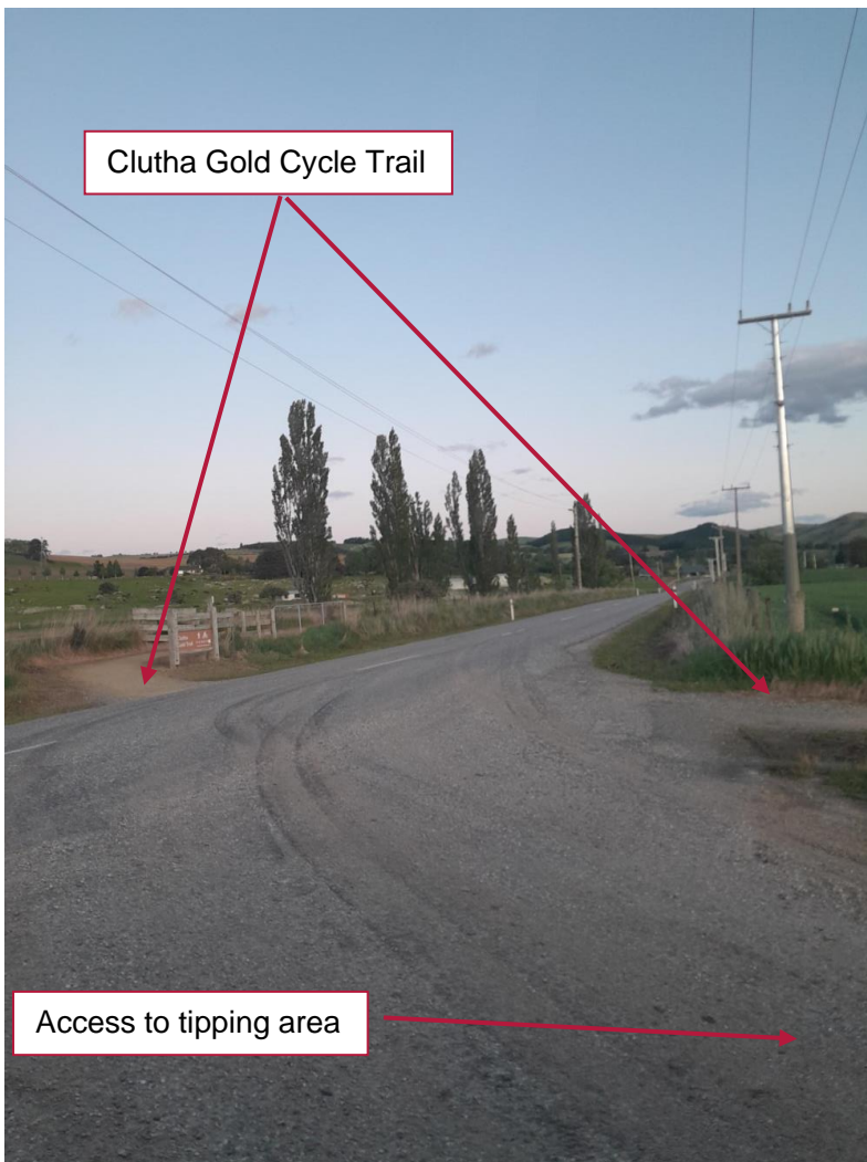
Figure 2.2 Photograph showing Clutha Gold Cycle Trail Crossing
