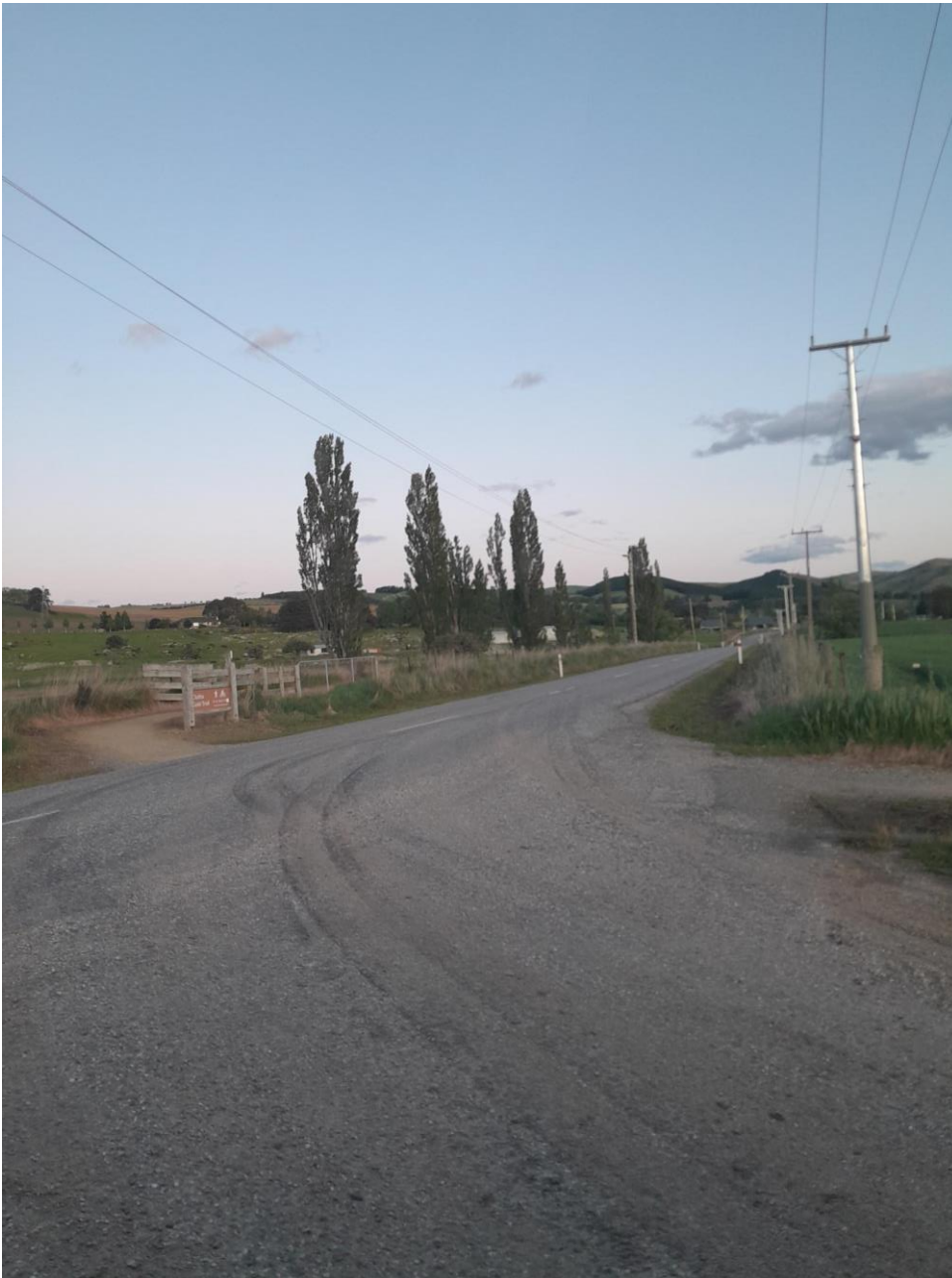
Figure 4.2 Looking south-east from southern access
