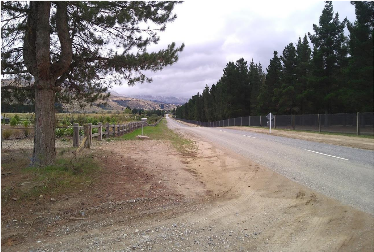
Figure 17: View north along Sandflat Rd from site entrance, looking towards Highlands Motorsport Park (obscured in distance).
