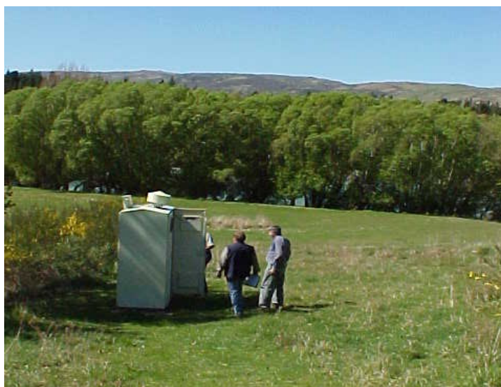
Bore control and bore site
