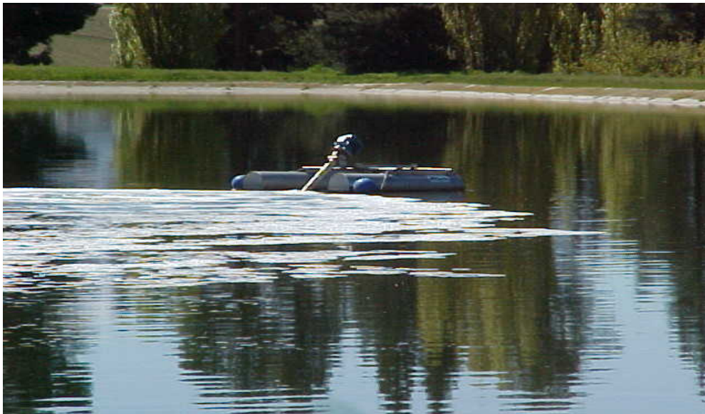
Aerator operating in Oxidation ponds
