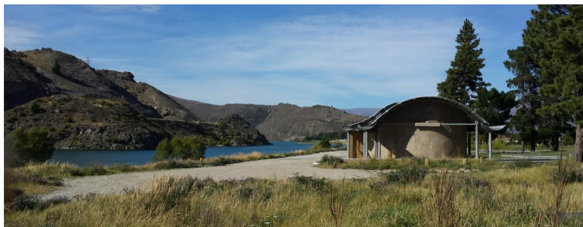
Cromwell water treatment plant- located on Alpha Street Reserve
