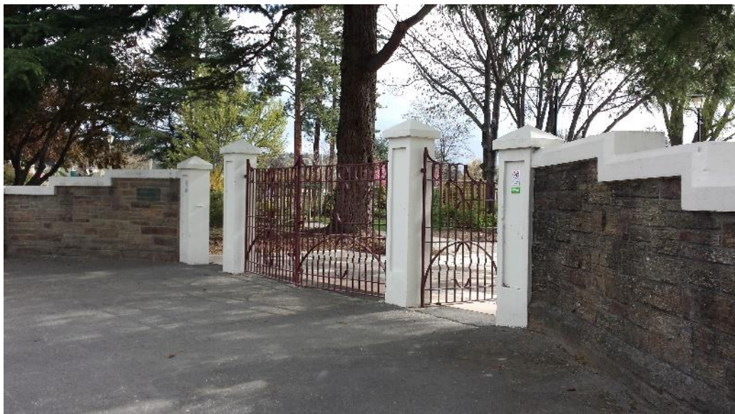
Tarbert Street entrance gates
