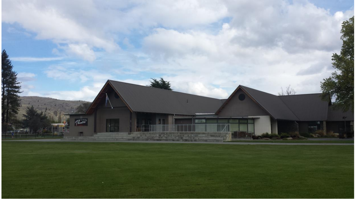
North East view of building
