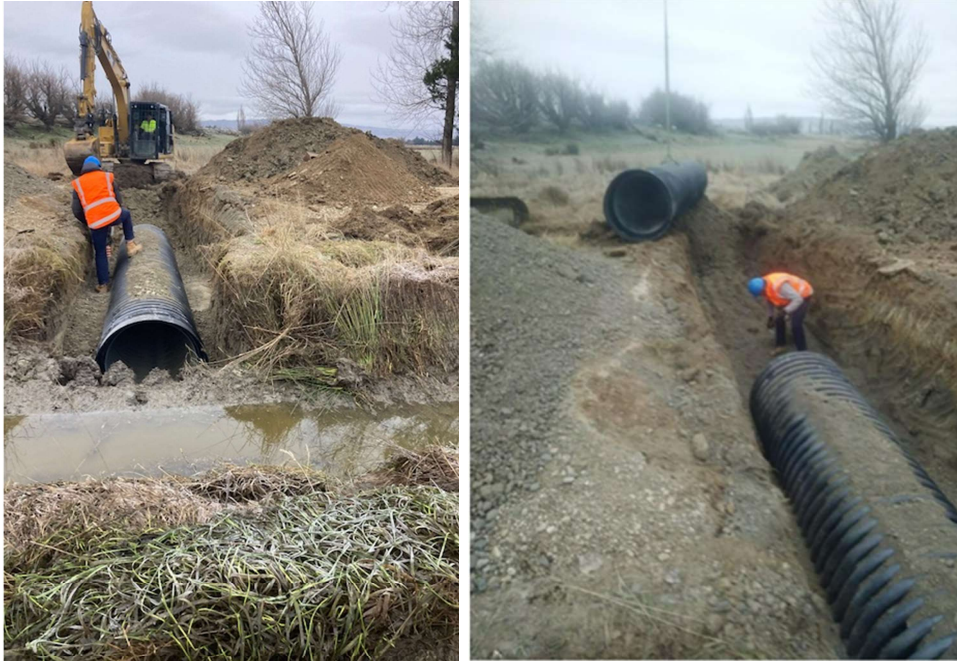
Figure 12: Installing a New 800mm Culvert on Wallington Road
