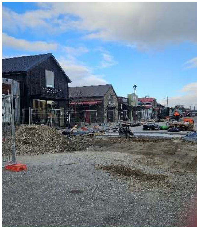
Figure 16: Holloway Street Clyde- Upgrade works
