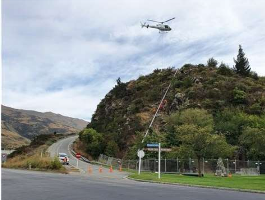
Figure 5: Helicopter working near the pipeline
