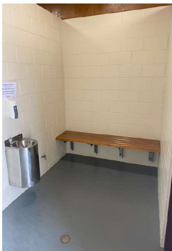
Figure 224: Before new toilet installation
