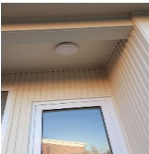
Figure 29: New LED button light units fitted both externally and internally.
