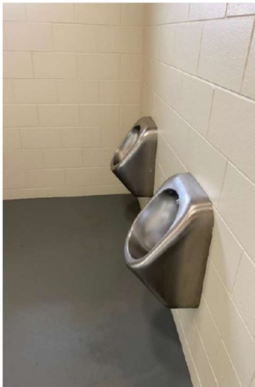
Figure 22: Inside men's Old Cromwell toilets - before new toilet installation
