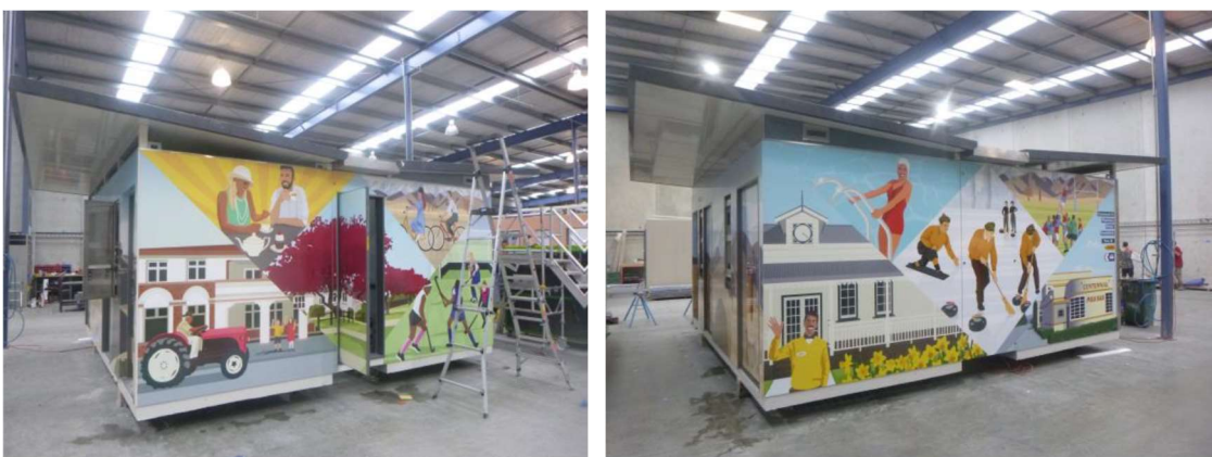
Figure 20: Toilet Block – post-production at the factory – artwork specific to Ranfurlly reflecting the art deco heritage.
