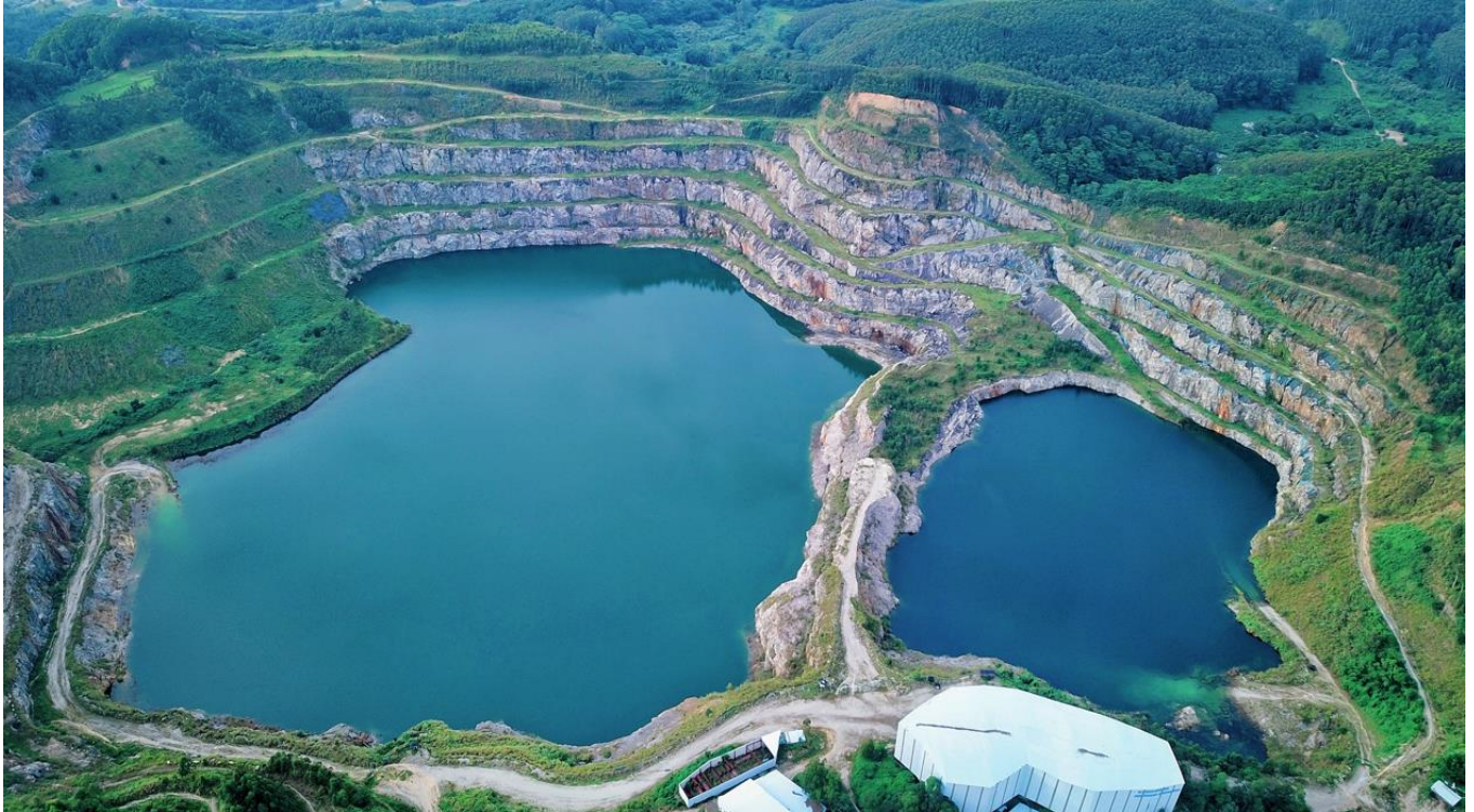
Figure 5: Guangzhou Pumped Storage Station (Source: Kong et al., 2017)
