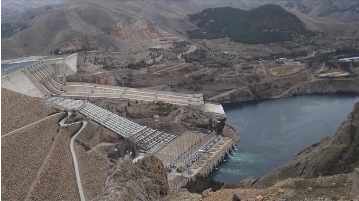
Figure 7: Norway Pumped Hydropower Dam (Source: Harby et al., 2013)
