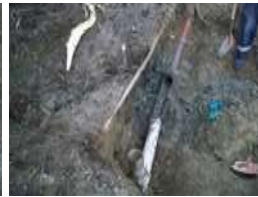
Inadequate jointing
