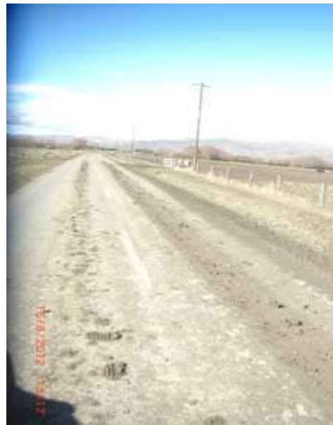
Mud tracked on Gimmerburn Waipiata Road
