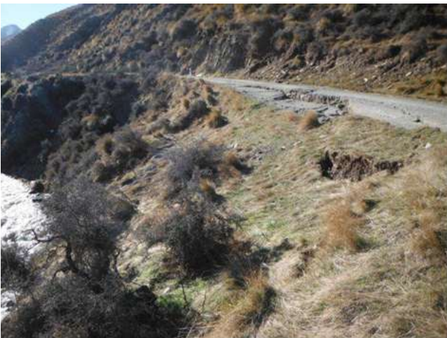
Danseys Pass Road Slip
