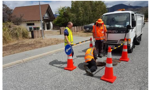
Drain View in action at Kirtle Place Cromwell
