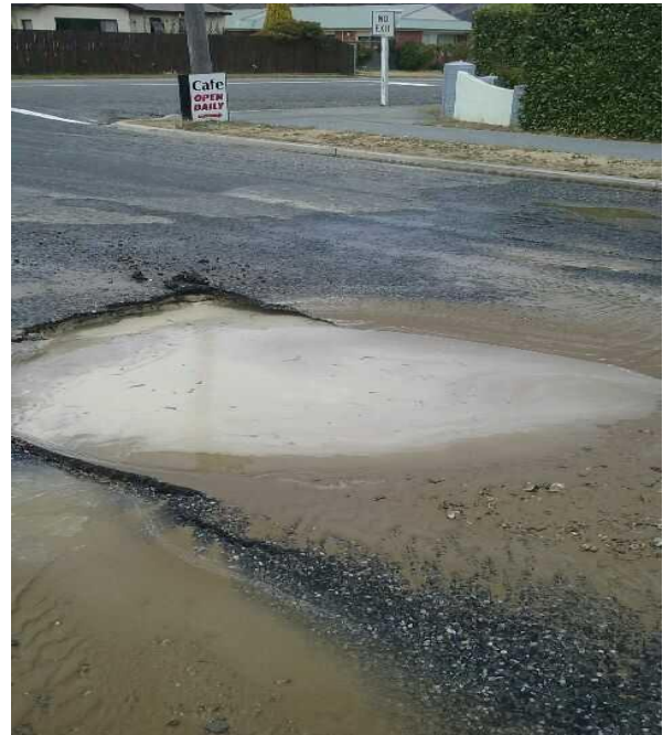
Prior to starting work
