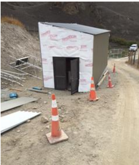
Partially completed ultraviolet disinfection building
