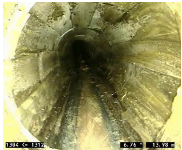
Wooden stormwater pipe
