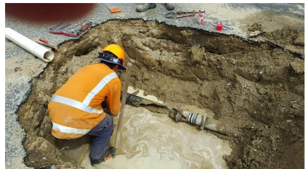
The main under repair
