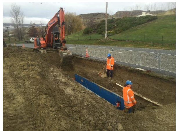
Cage protected excavation on Felton Road drainage improvement
