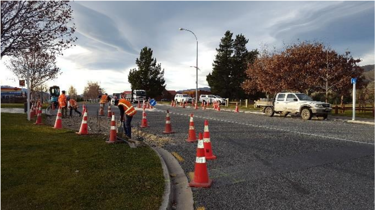
Fulton Hogan staff working on Cromwell pedestrian crossing Safety Improvement project.
