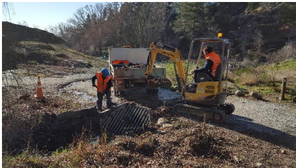
Stormwater Grate in Gillaly Way, Alexandra.
