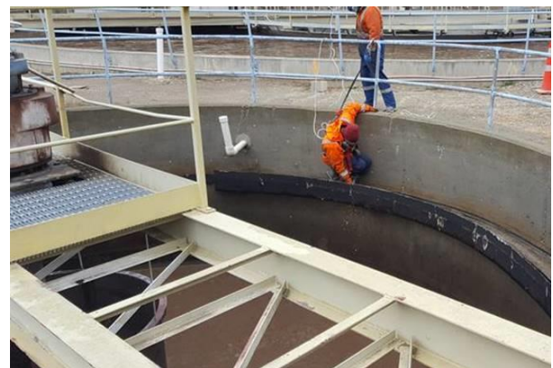
Removal of the old weir in the sludge thickener.
