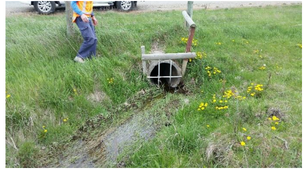
Perry Street Ranfurly pipe inspection.
