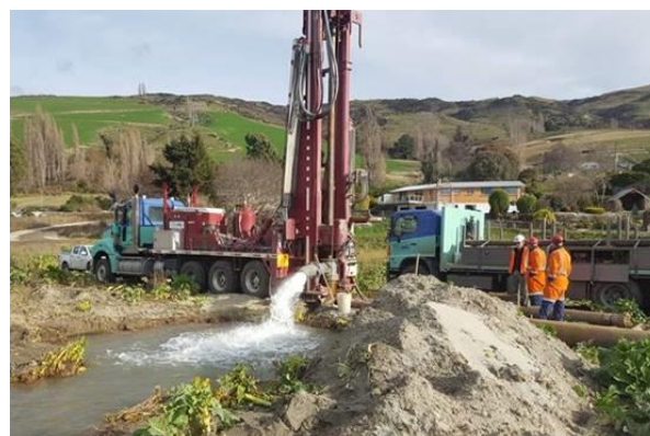
Drilling of the new bore
