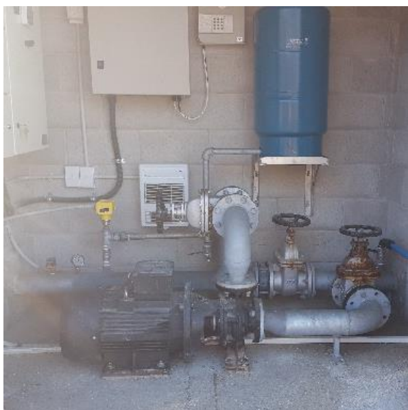
Old booster pump station.
