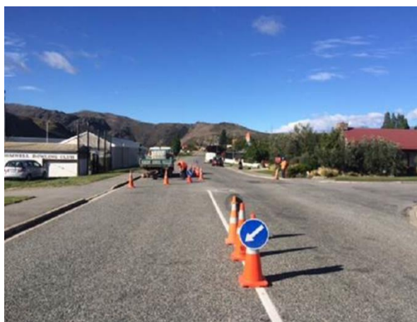
Fulton Hogan carrying out pre-reseal pavement repairs in Cromwell.
