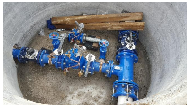
Pressure regulating valve.
