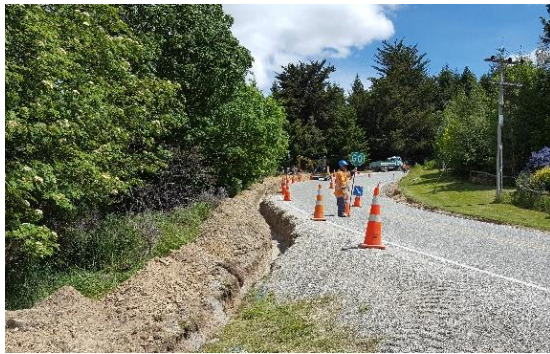
Trench for the new main next to the road.
