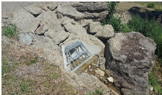
New outlet structure.
