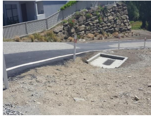
Improved road entrance and catchpit.
