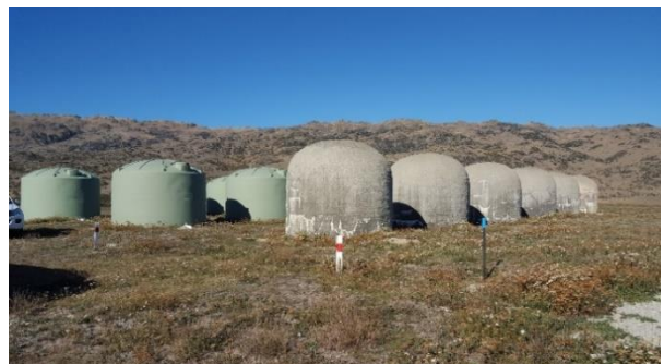
Old Concrete tanks to be replaced.
