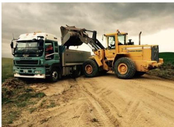
Surface water channel upgrading work in progress.
