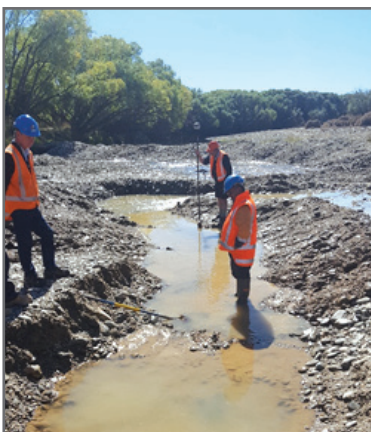
Exposing and checking inlet screen
