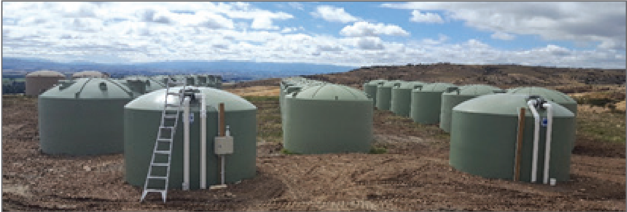
New tanks installed and connected
