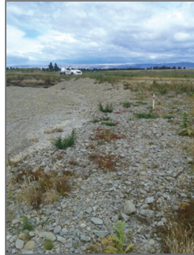
Pipe reinstated and river redirected
