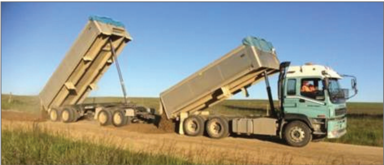
Re-metalling underway on a Maniototo road
