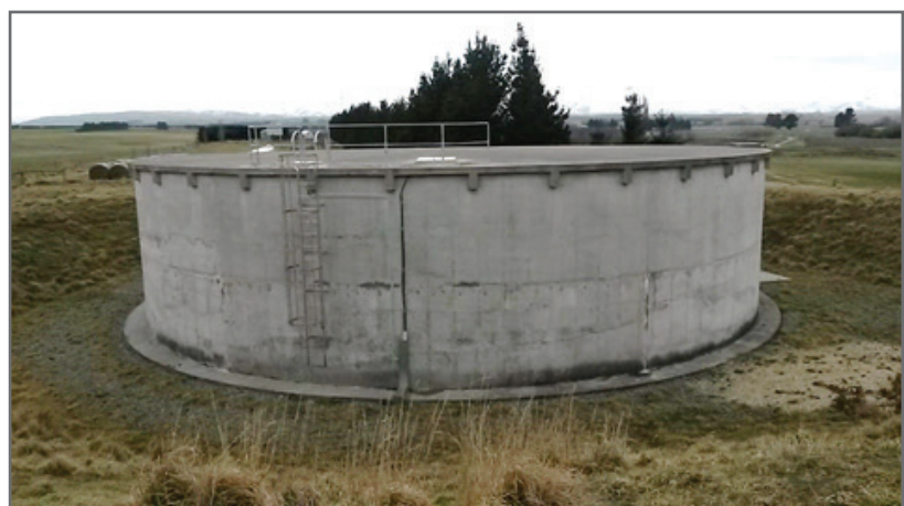
Ranfurlly Water Reservoir
