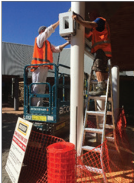
The new metal support frame work installed
