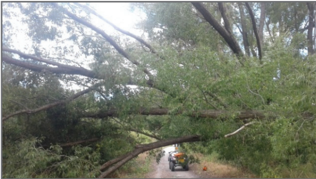
Asplundh completed vegetation clearance along the length of the Alexandra to Clyde River Track with some sizeable windblown trees coming down.
