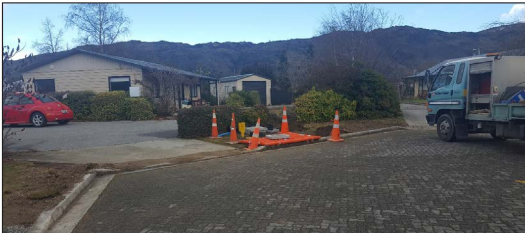
The Whistlestop water main renewal.
