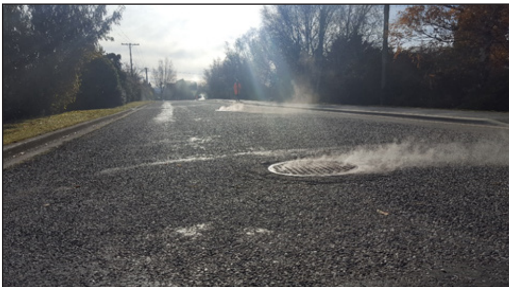
Smoke escaping from manholes in the street.
