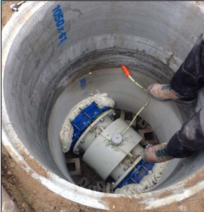
Installation of Flow Meter during construction.
