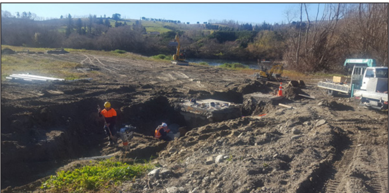
Bore site during construction and pipe connections in progress.
