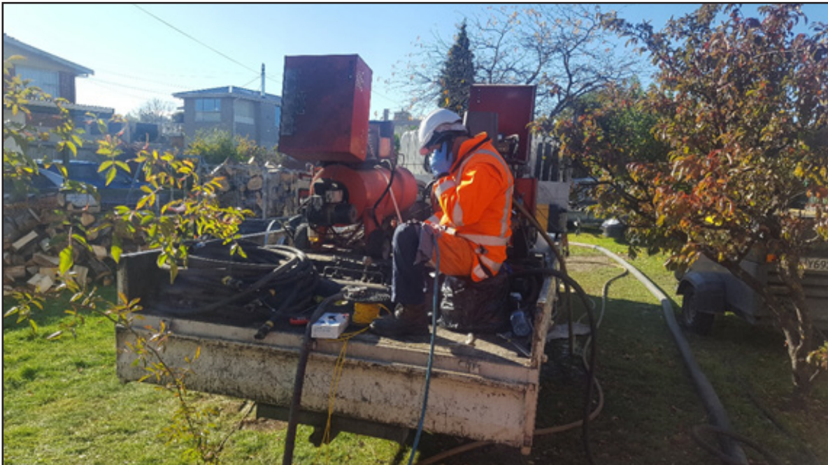
Relining operator and equipment truck.
