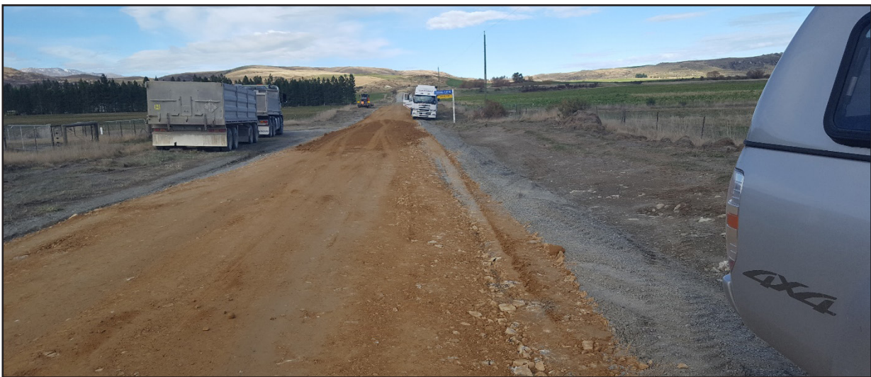
Re-metalling on St Bathans Loop Road.
