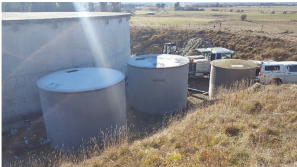
New bypass tanks in place
