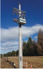
New Transformer for Power Supply
