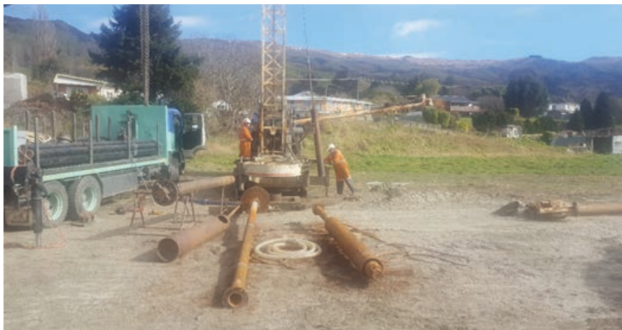
Drilling crew on-site to redevelop bore 2
