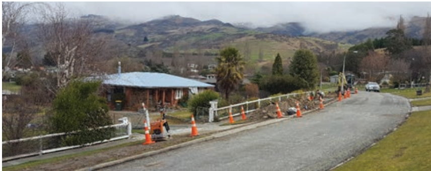
Tamblyn Drive during the water main renewal works
