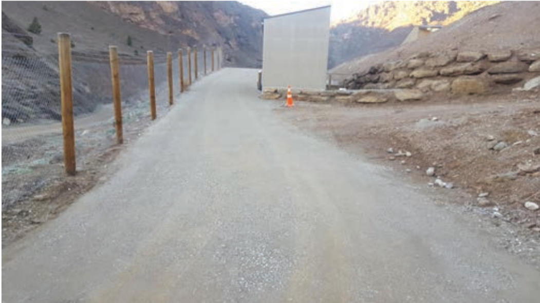
Formed entrance road in a much better condition
