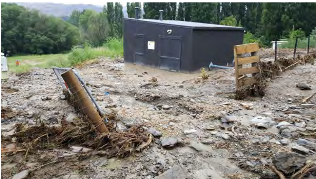
Roxburgh water treatment plant after the rain event.
