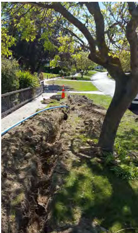
Rider main being installed in Tamblin Drive, Roxburgh.
