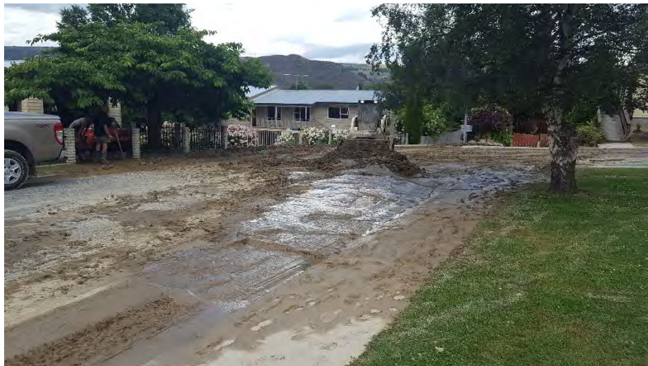
Loader clearing silt in Paisley Place, Roxburgh
