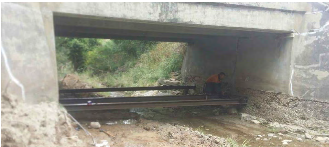
St Bathans Loop Road temporary props
