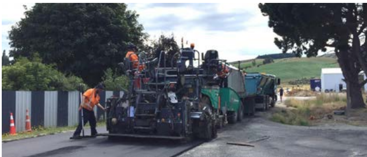
Asphalt resurfacing on School Road, Millers Flat
