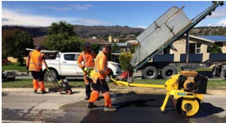
Asphalt levelling in preparation for resealing
