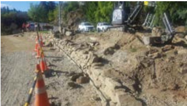
Block wall being repaired.
