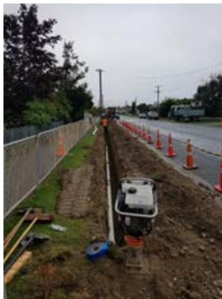
Watermain renewal on Bantry Street.
