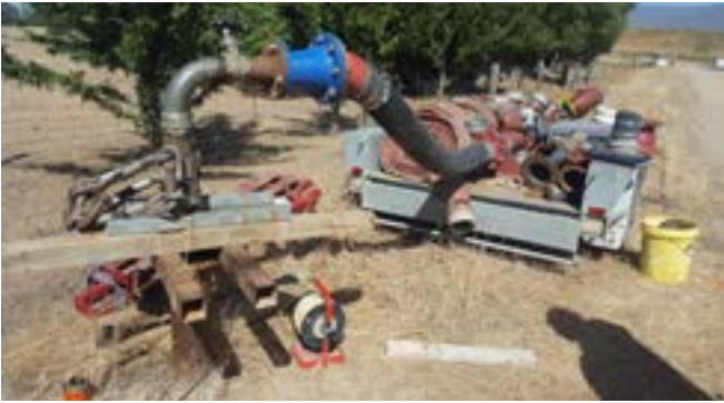
Bore test pump installed and operating on the existing bore.
