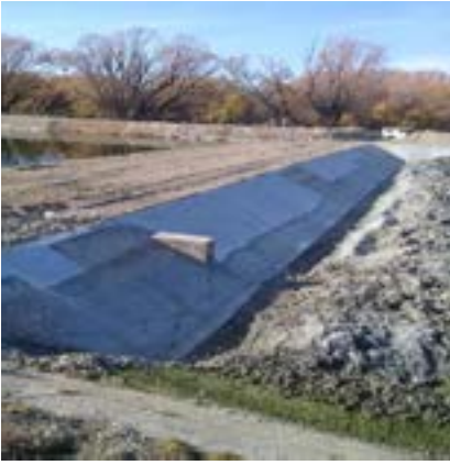
Repaired wave band in Pond 2
