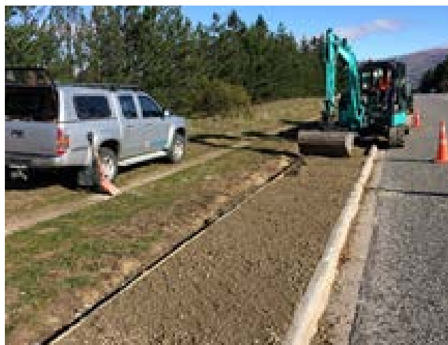
Footpath construction - Barry Ave (Butchers Drive to Richards Beach Road)
