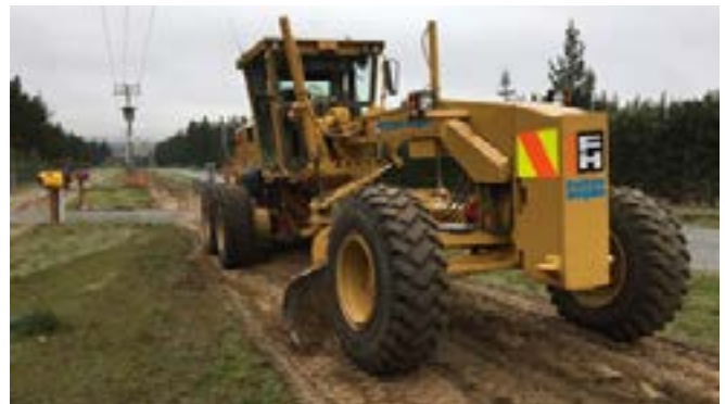
Grader shaping the cycleway on Bannockburn Road
