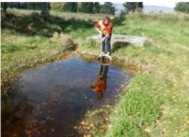
Clearing a blocked stormwater inlet grate
