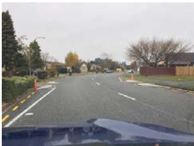
Pedestrian crossing point kerb build-outs - Waenga Drive, Cromwell
