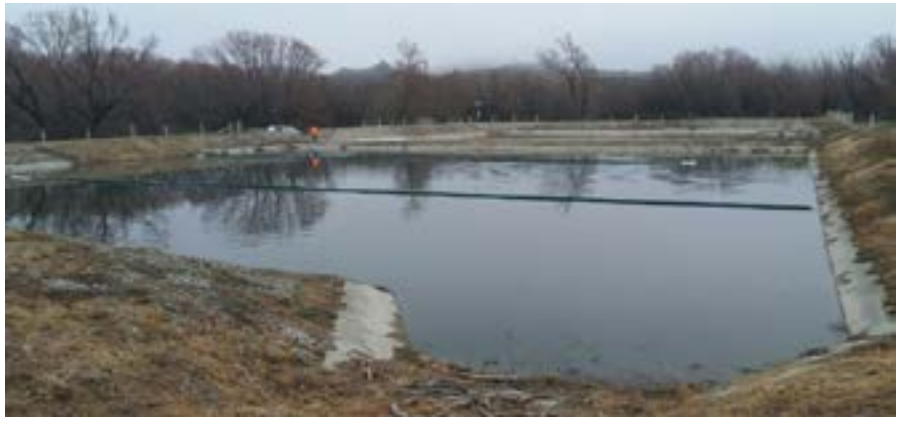
Baffles installed on Pond 1
