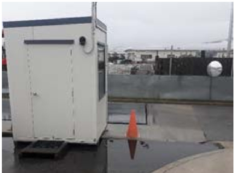
Flooding at the Cromwell Transfer Station weighbridge
