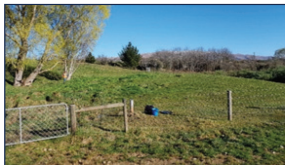
Ettrick Closed Landfill
