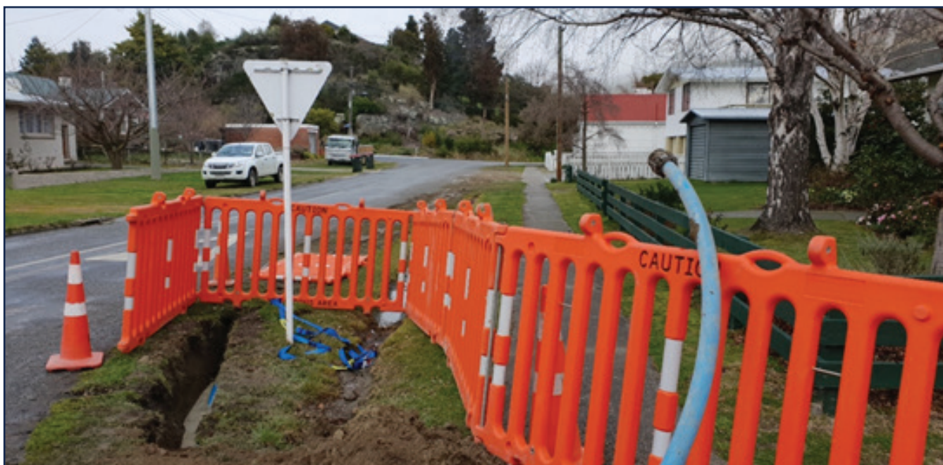
Meter separations being undertaken on Hermitage Street
