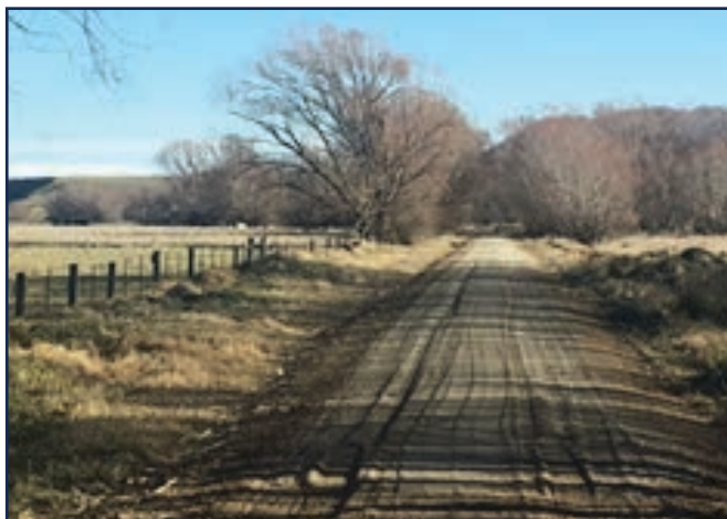
Freeze thaw conditions – Auripo Road – August 2018
