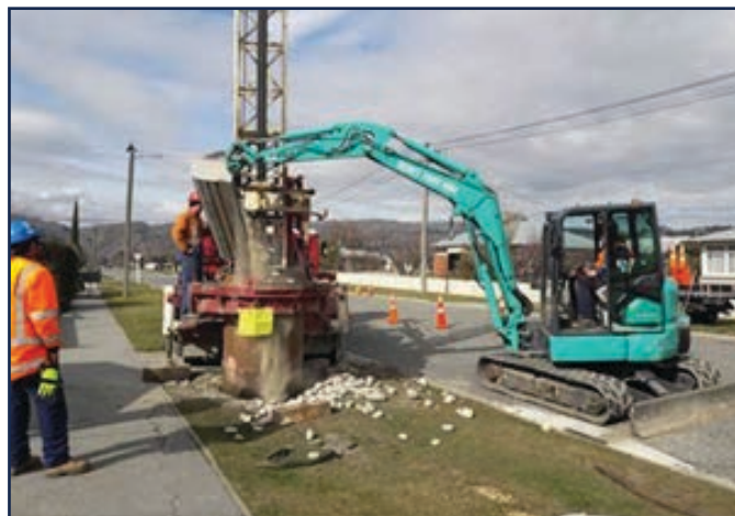
Ventry Street soakpit installation – September 2018
