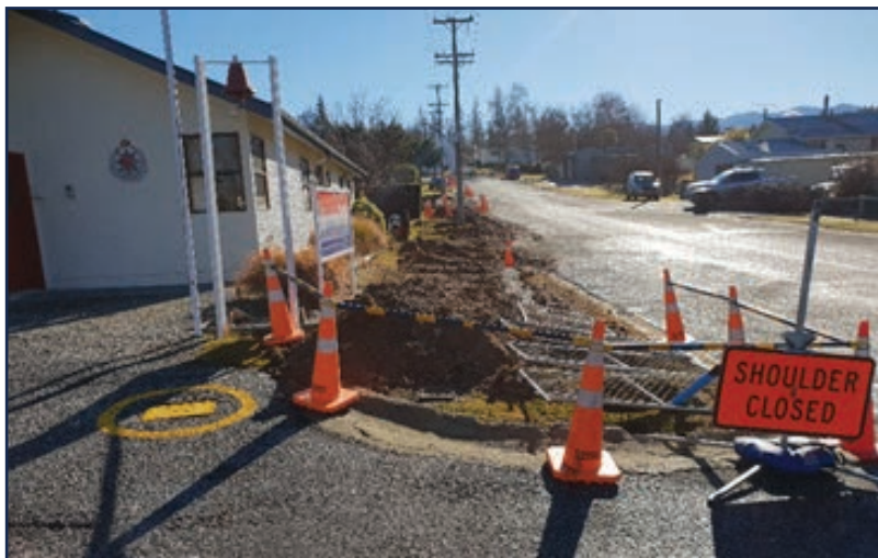
Excavation on Tay St, Naseby
