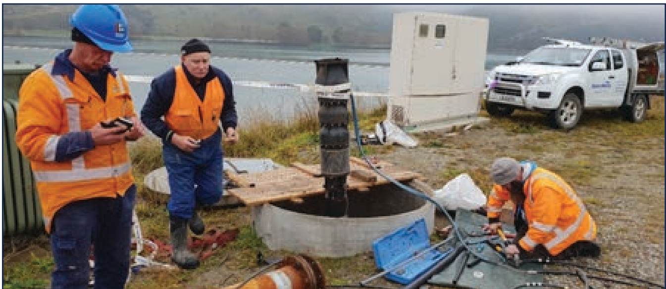
Connecting the spare pump
