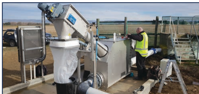
New screen being commissioned in Ranfurly by the supplier
