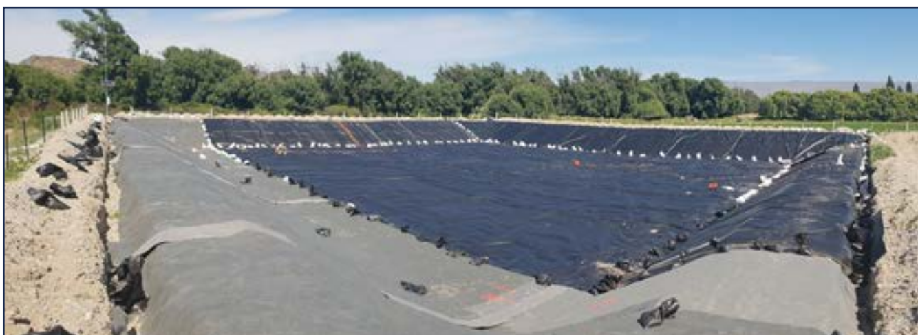
Image of Pond 2 during the installation of the liner.
