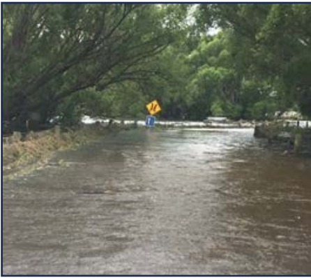
Maniototo Road - Flooding of the Taieri River at Halls Ford bridge
