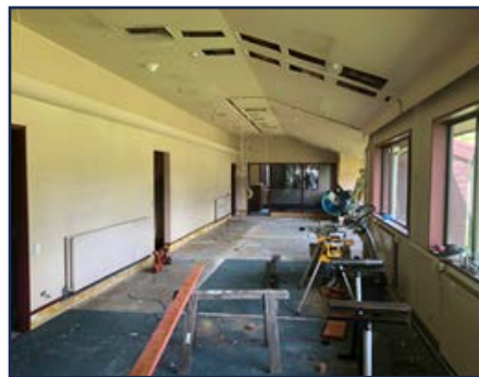
The refurbishment in progress.
