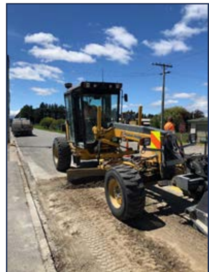
Grading on Pery Street, Ranfurly – pre-reseal repairs
