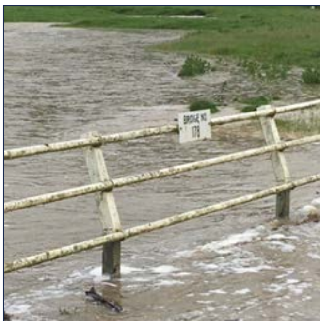
Tima Burn Road – Oven Hill Creek flooding at Bridge 178
