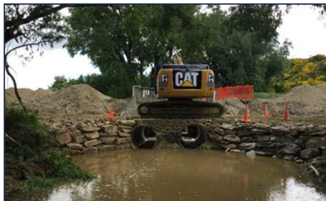
Temporary road crossing and culvert at Bridge 94, St Bathans Loop
