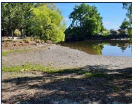
Lanes Dam water levels at 8 November 2018
