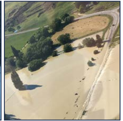
Ida Valley-Omakau Road – flooding of the Manuherikia River requiring full road closure
