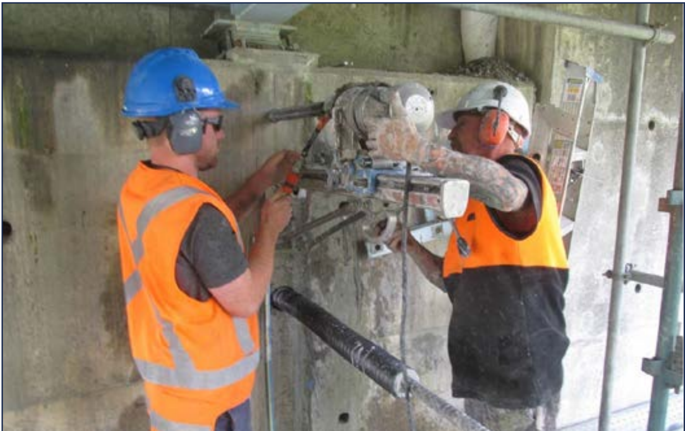
Subcontractors undertaking drilling of seismic linkage bar holes at Jedburgh Bridge
