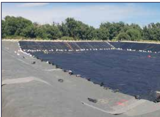
Pond two during the lining process.
