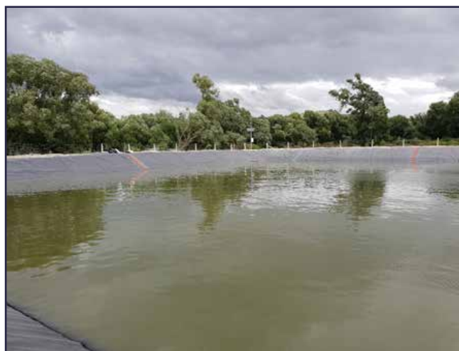
Pond two completed and back to normal operation.
