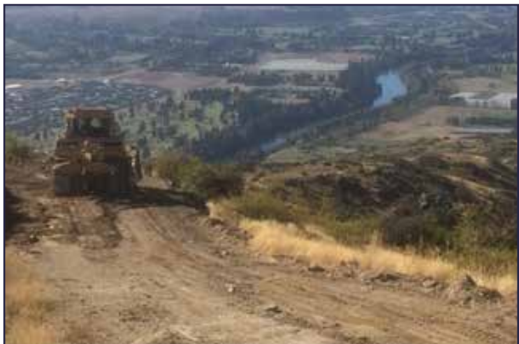
Shaping and preparing Hawksburn Road for gravel
