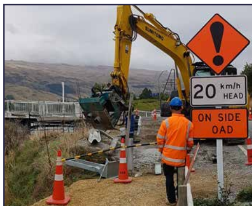
Guardrail realignment Jedburgh St Bridge
