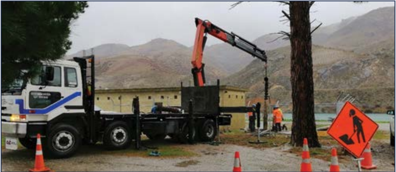
Cromwell booster pumps being lifted for inspection.
