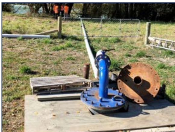
Roxburgh Bore 1 pumping to the river.
