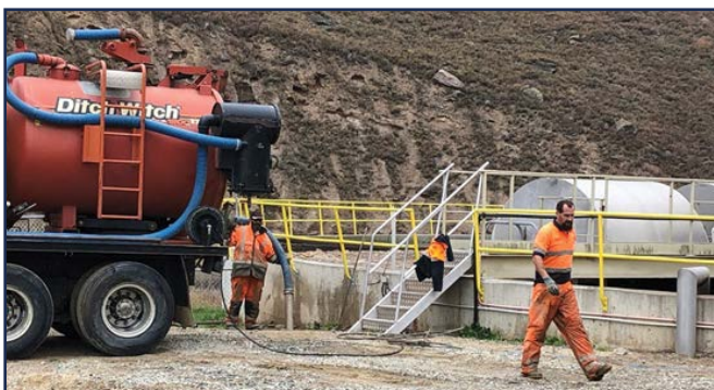
Hydro excavation works at the Alexandra wastewater treatment plant.
