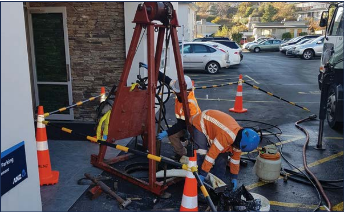
Installation of the liner being completed.
