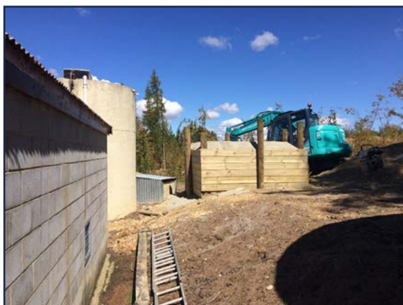
Hard stand for the relocation of the mixing tank.
