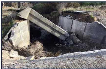
Demolition of Bridge 94 – St Bathans Loop Road, May 2019.
