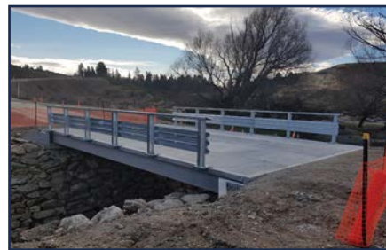
New Bridge 94 almost complete, St Bathans Loop Road - July 2019.
