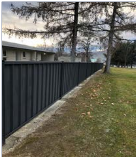
New fence between Goodger Court and the Reserve
