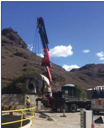
Removal of the old inlet screen.
