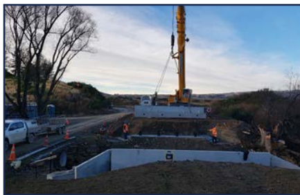
Installation of the new Bridge 94, St Bathans Loop Road, June 2019.
