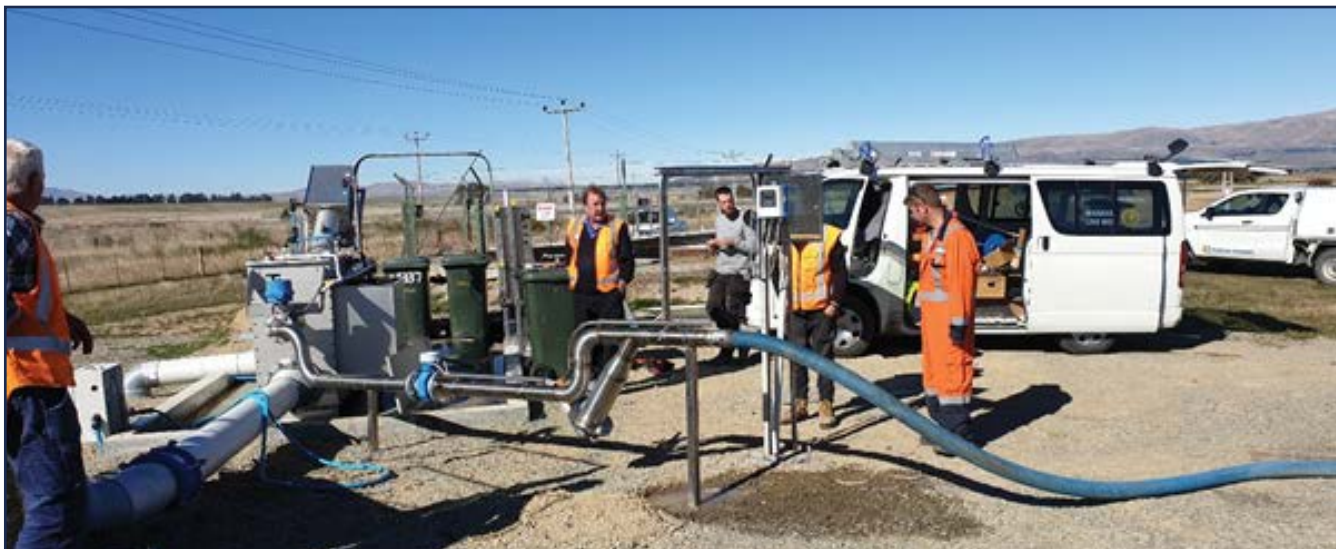
Testing the septage connection system.
