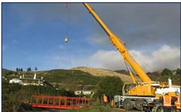
Tweed Street foot bridge, Roxburgh, June 2019
