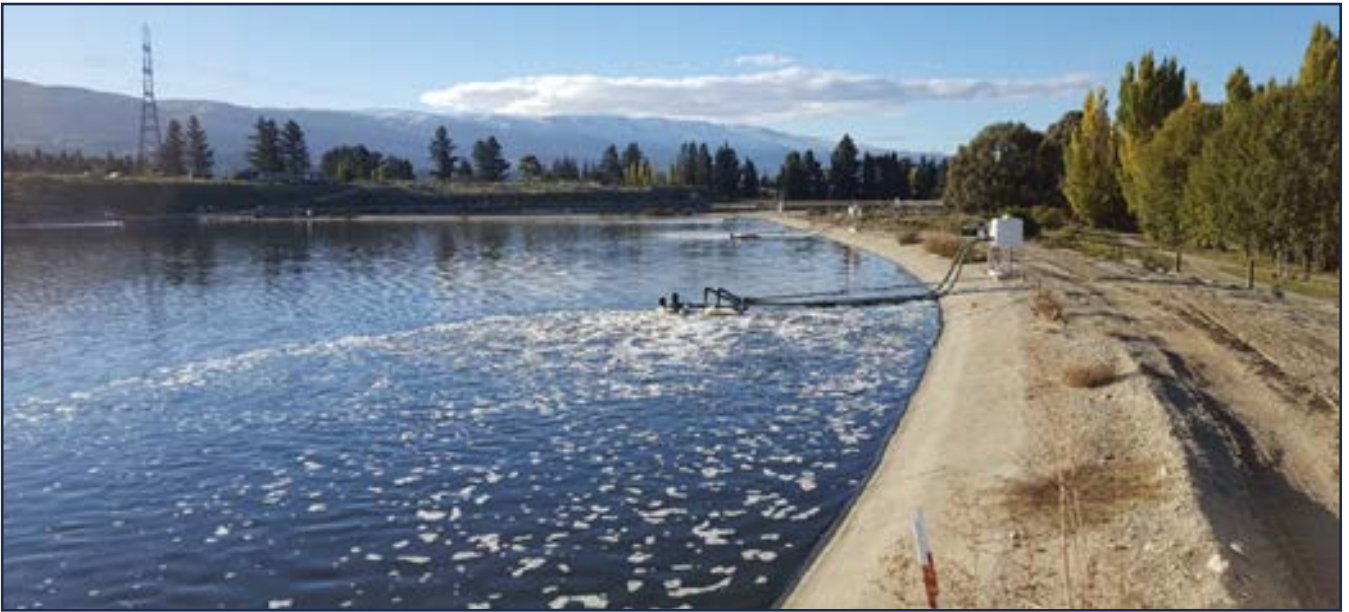
Aerators on Cromwell oxidation ponds
