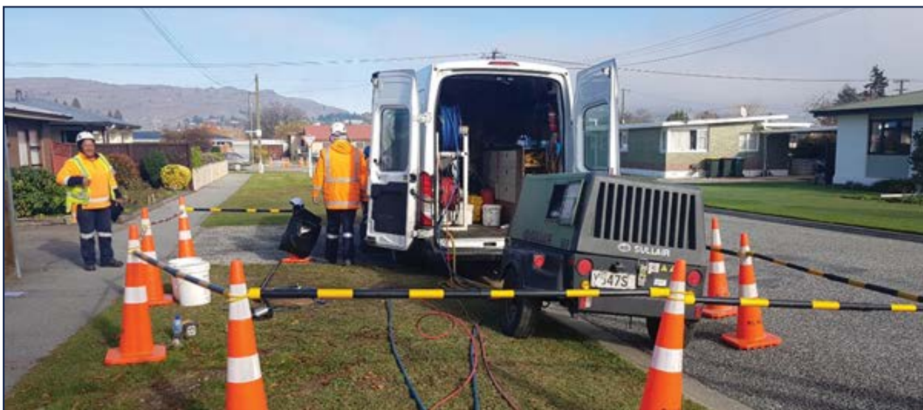
CCTV video inspections prior to the relining work.
