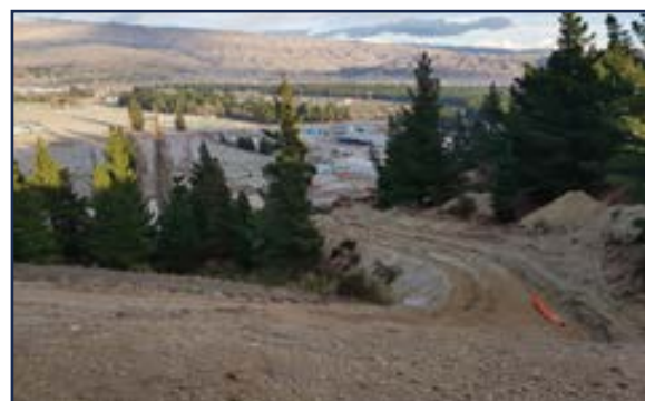
Pipeline route to the Northern Reservoir.
