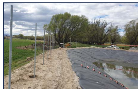
New fence being installed at the Omakau Wastewater Ponds.
