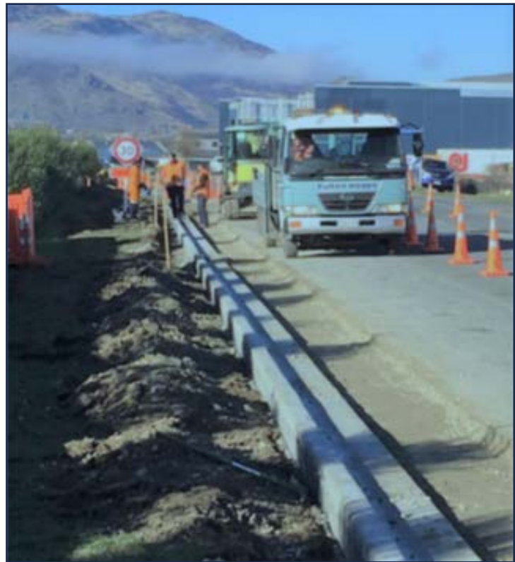
Reinstating kerb, McNulty Road – July 2019
