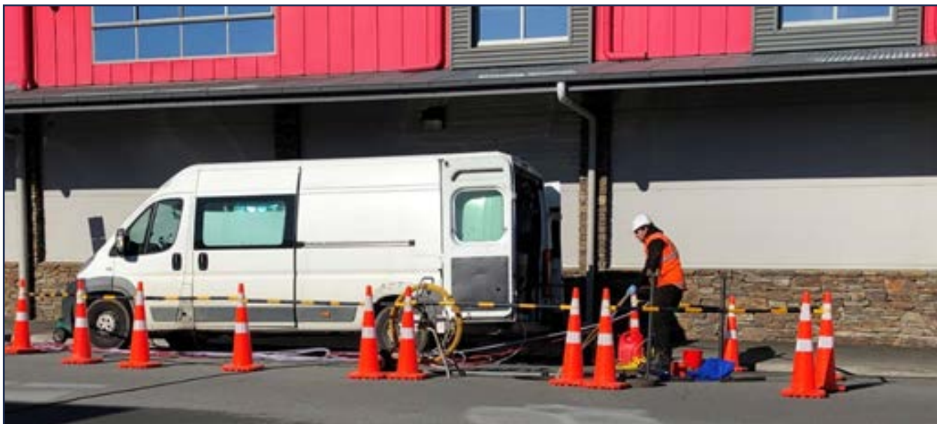
Smoke testing contractor on site.
