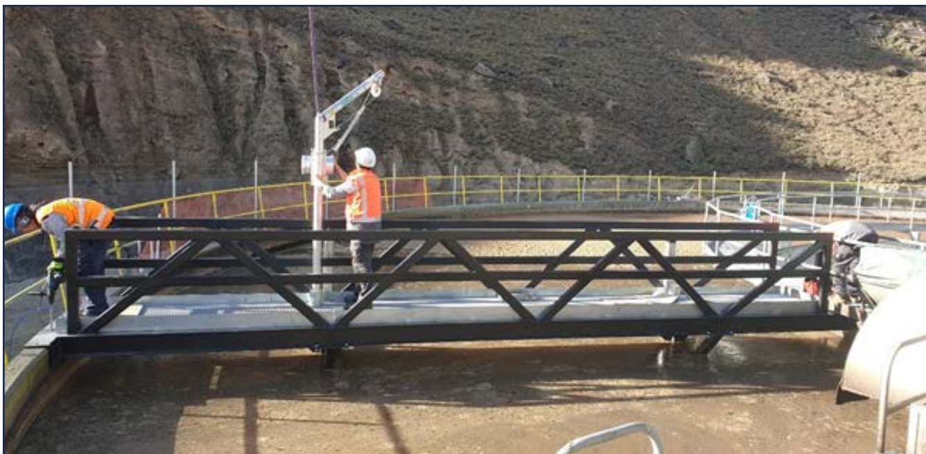
New bridge being installed over the aeration ditch.
