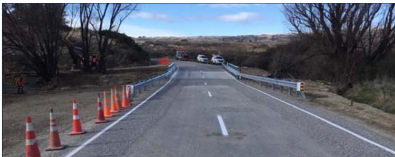
Bridge 94 completed, St Bathans Loop Road - July 2019
