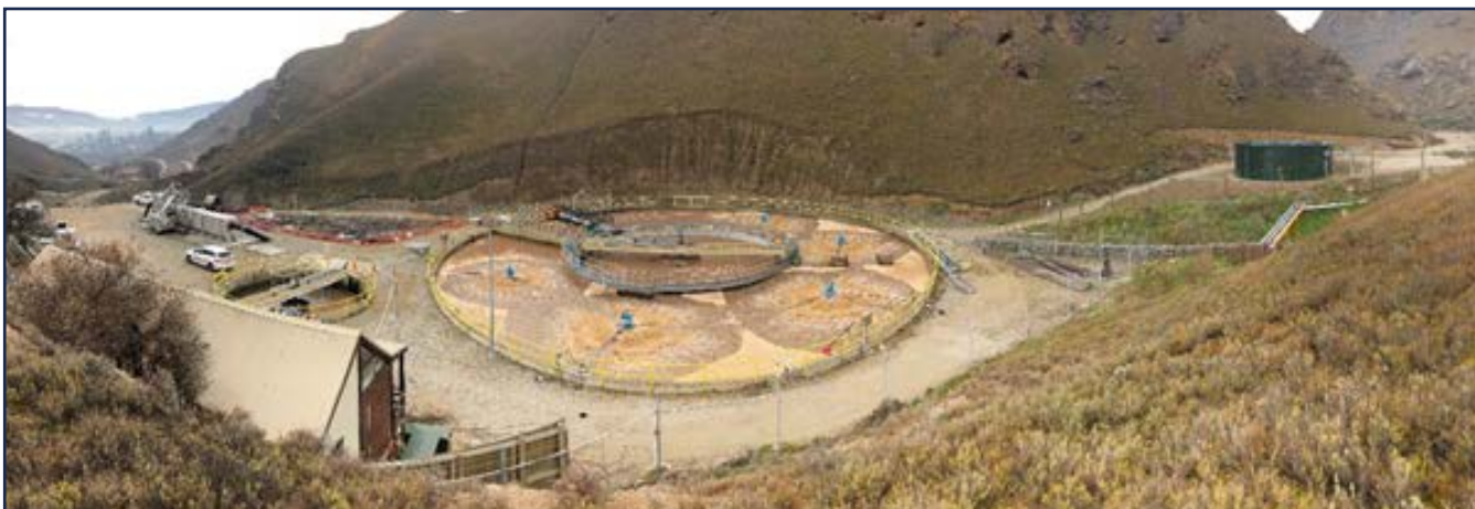
View of the Alexandra Wastewater Treatment Plant site with all aerators running.
