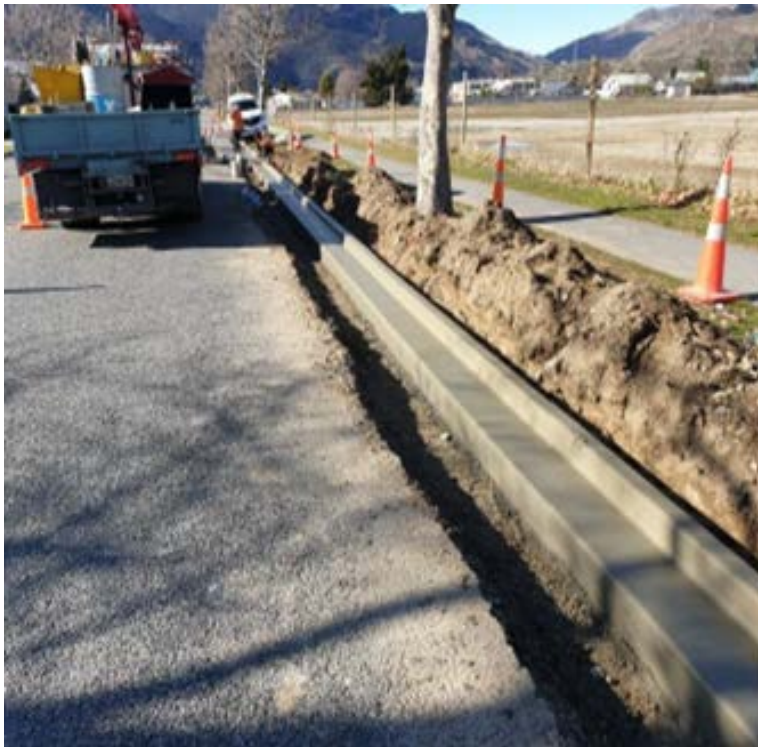
New kerb and channel, Gair Ave
