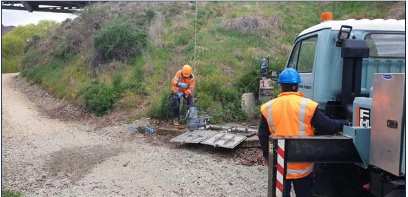
New pump being lowered into the pump station.
