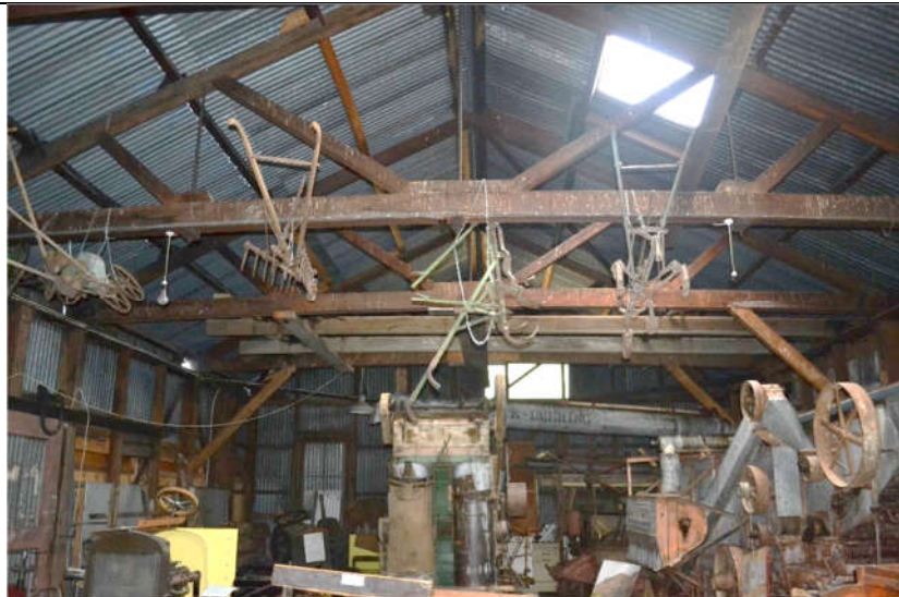
The trussed roof frame of the Shed – the bottom chords appear to deflect
