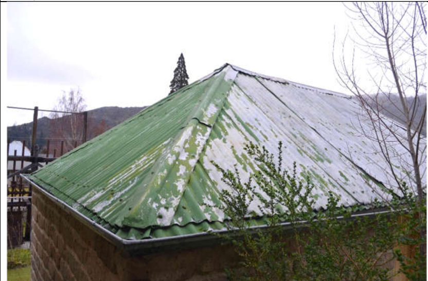
Building H: Dairy roof
