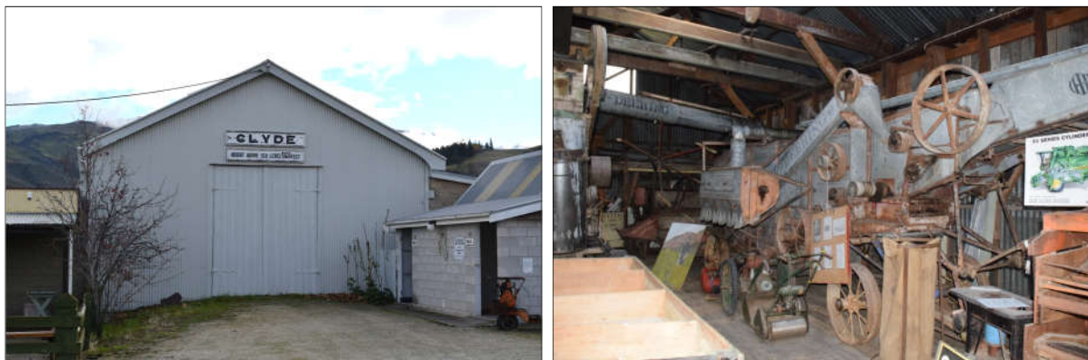
Figure 7: The front, south-east end of the Goods Sheds (left) and a view of the interior, looking west (right).
