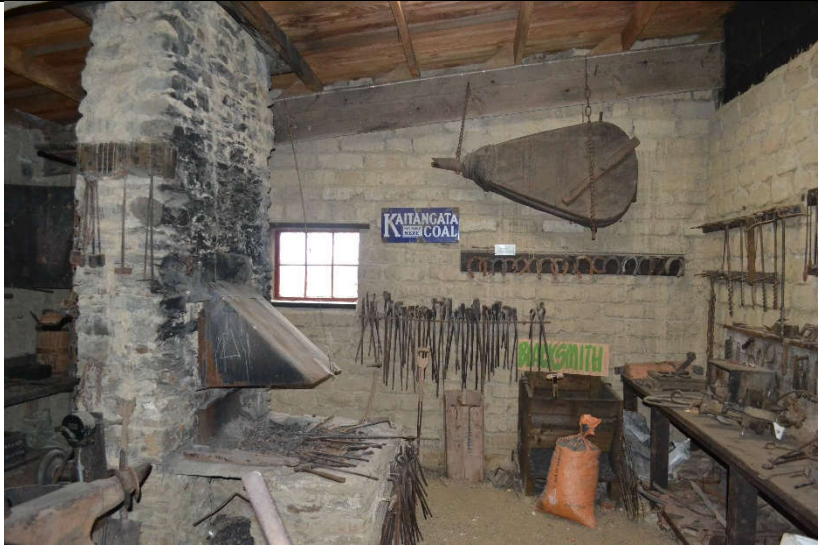
Unrestrained schist chimney stack
