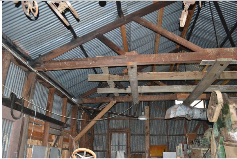
Missing strut and slack steel tie to the bottom chord in the foreground
