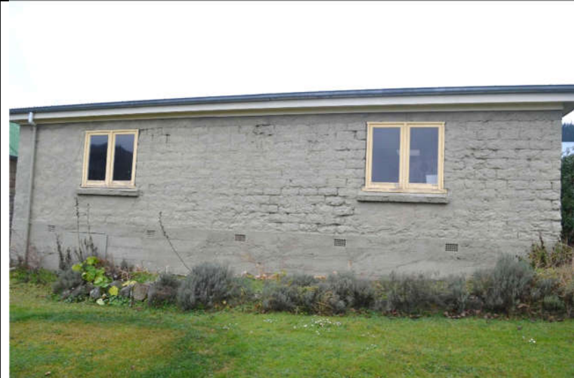
Building G – Painted mud brick south wall Dairy, Toilet Block, Meat Safe
