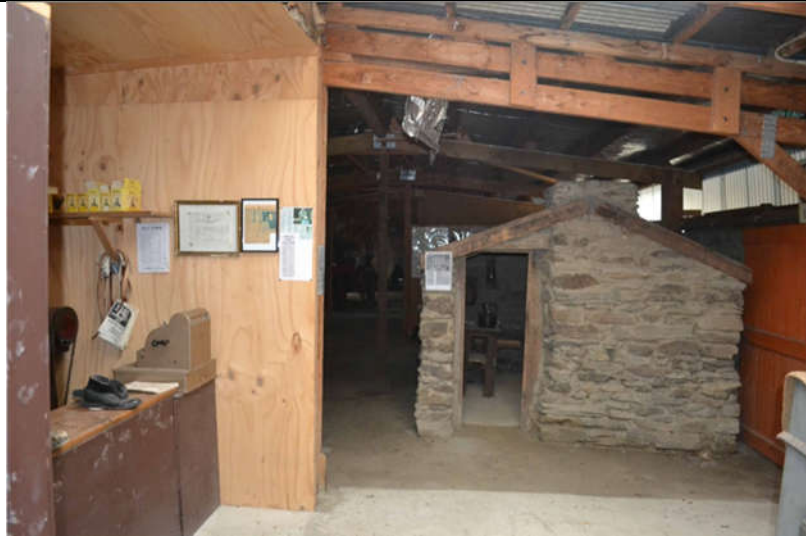
Looking East within the rear part of the building
