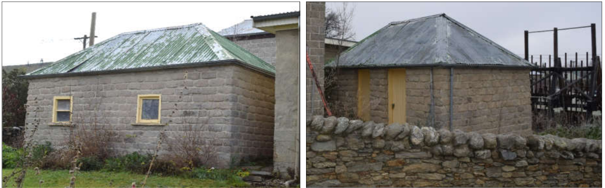
Figure 14: The Dairy building south-west facing exterior (left) and the north-facing exterior (right) with the stamper battery in view in the background.
