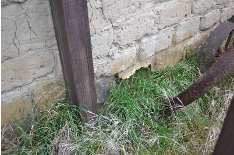
An example of mud brick decay at ground level
