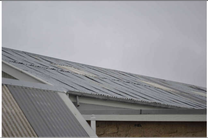
Lifting of roofing sheets to the north slope
