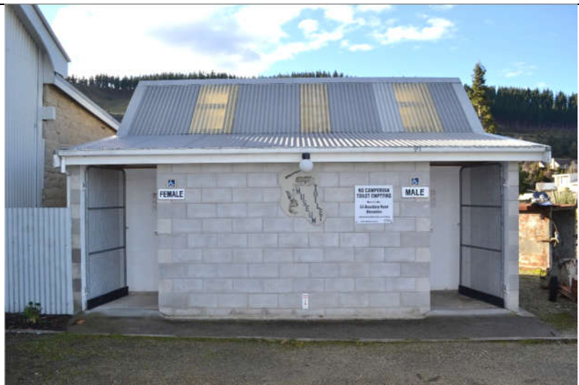
Building E: Modern Toilet block
