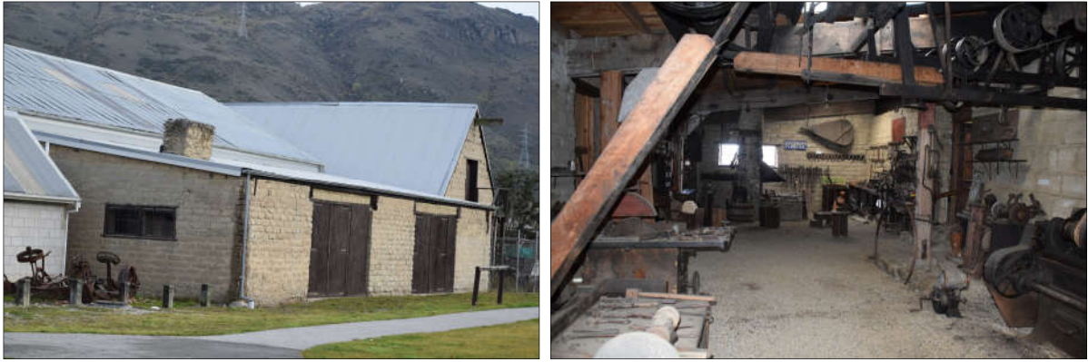
Figure 8: The Blacksmiths building exterior (left) and an interior view looking east (right).
