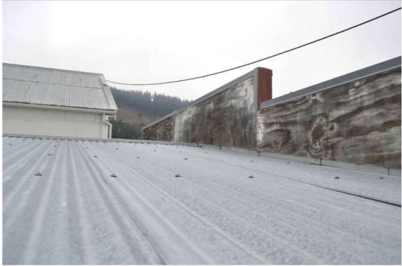
The rear face of the front parapet and adjacent roof
