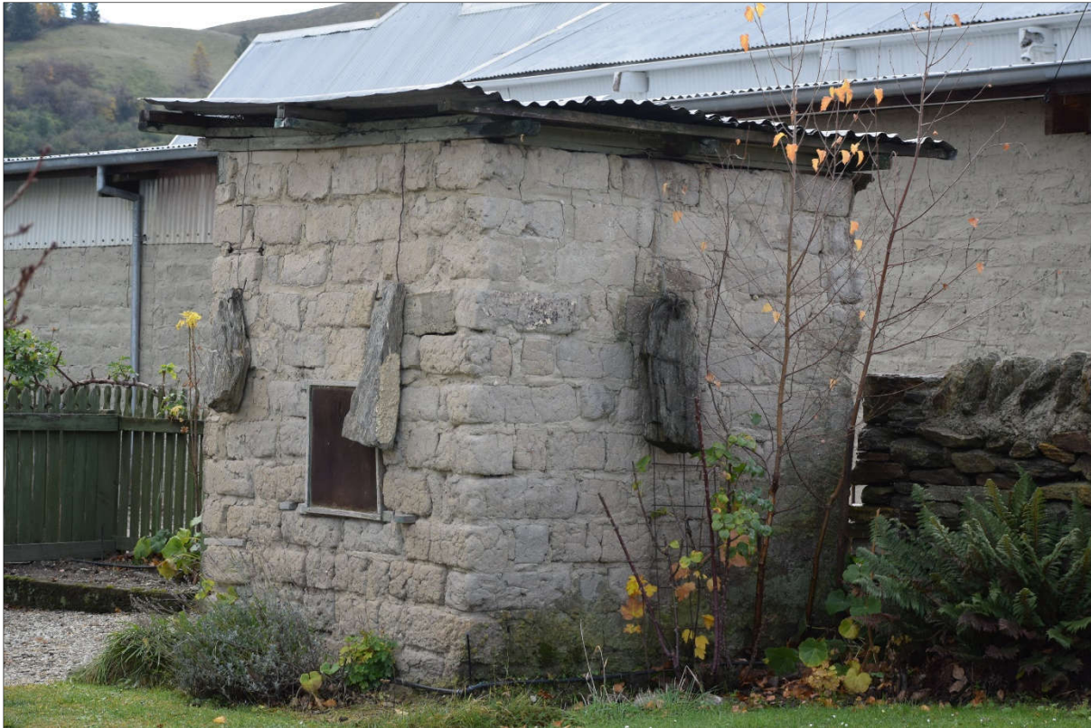
Figure 16: The meat safe structure to the south-east of Factory Building A.
