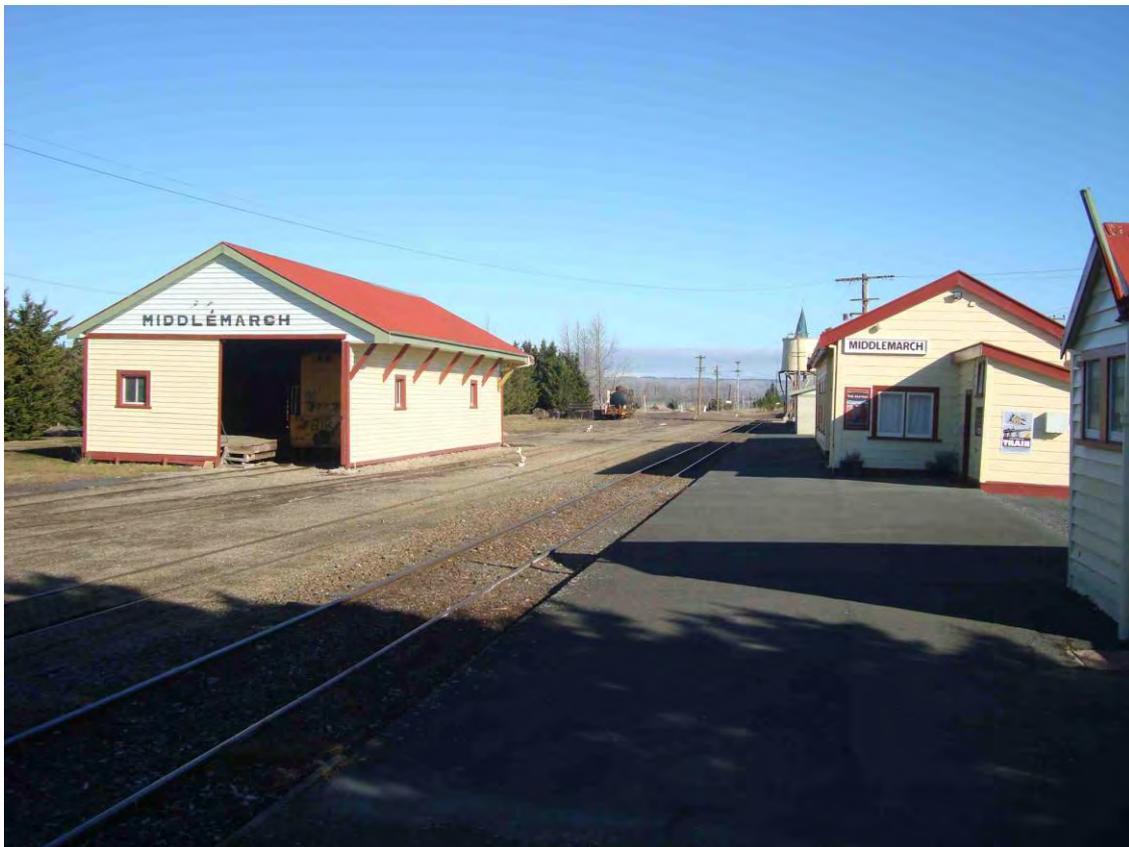
Figure 3: Middlemarch station and goods shed – opened 1891. It is a Type B station without a platform veranda.
