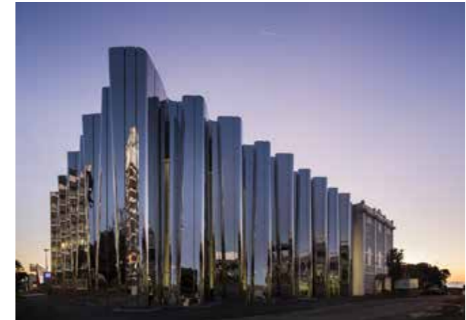
There is the potential for a landmark structure and private investment is encourage in visitor or hotel accommodation.
