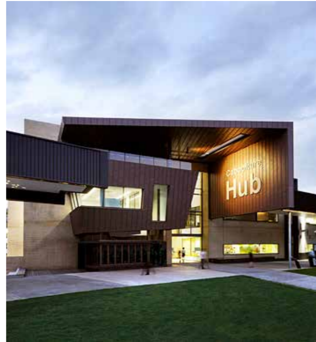
Opportunity for a new Civic building that includes a integrated library, resource centre and expanded administration spaces, as well as commercial tenancies (cafe, retail)
